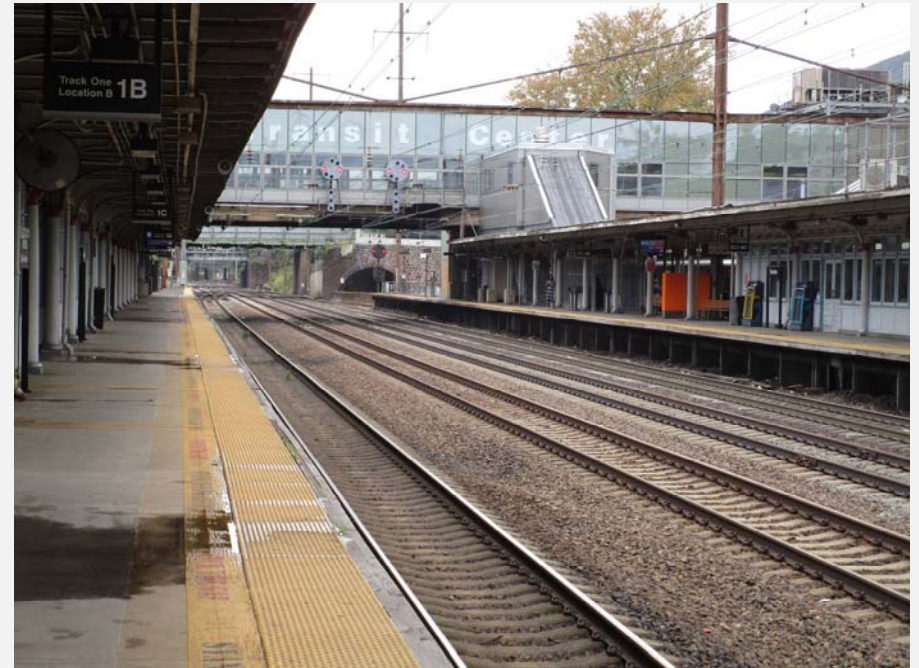
Looking west across center tracks towards westbound platform and Station's upper-level pedestrian concourse
