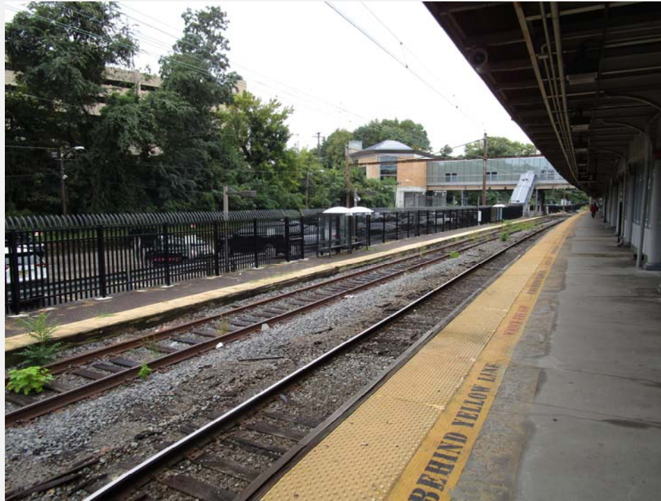
Looking west across eastbound tracks at existing low-level side platform
