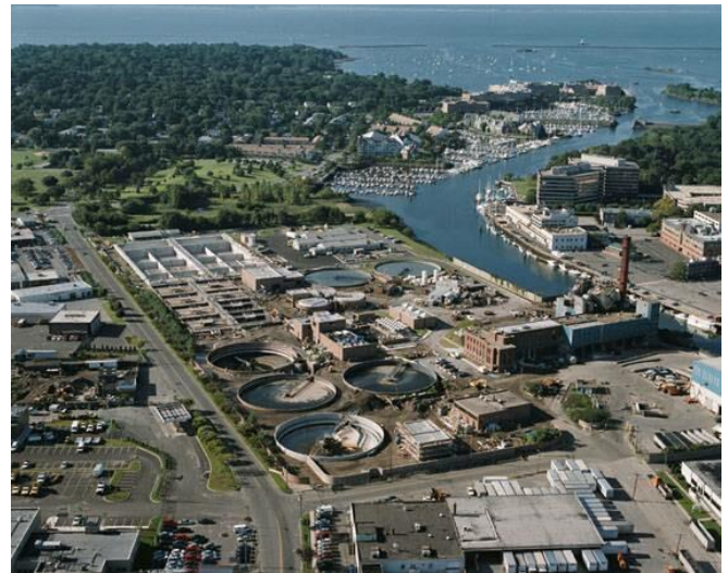
The Stamford (CT) Water Pollution Control Facility
