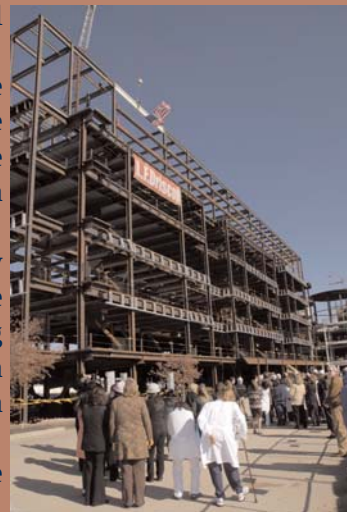
Construction site of the Meridian expansion funded by auction rate market vbonds that were issued in 2007 and converted in 2008
