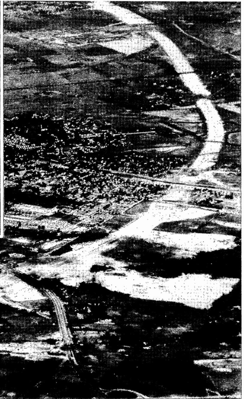
AIR PHOTO OF 6.55 MILE SECTION OF TURNPIKE Graded by New Jersey Highway Department from Route 4 Parkway to Morse's Creek. Inset shows graded portion of Route 35 interchange in more detail.
