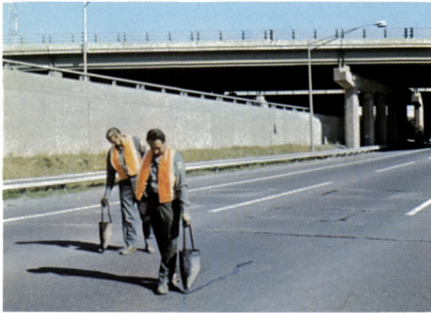
Sealing pavement cracks with tar bucket in Edison area.
