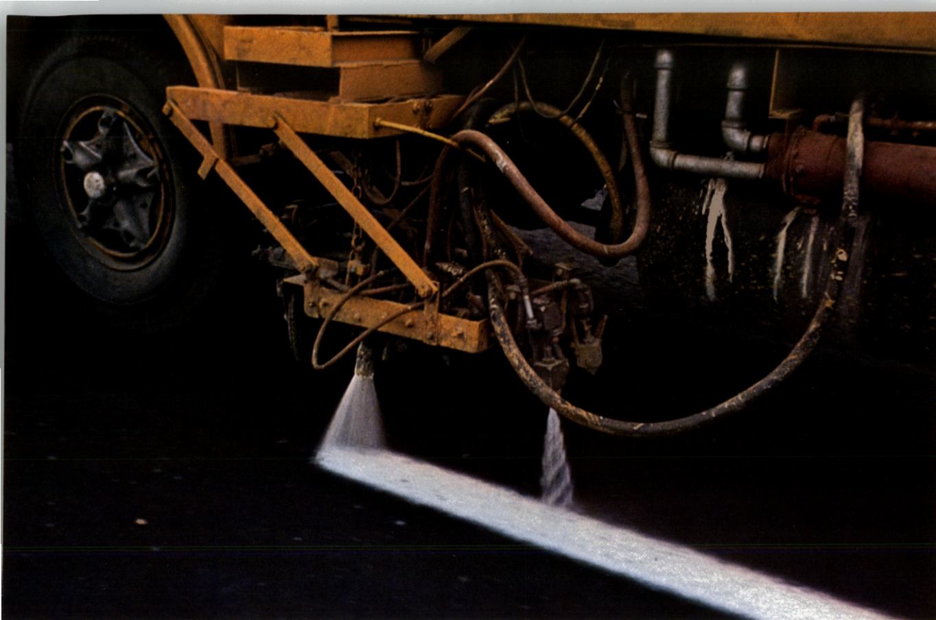
1200 miles of travel lanes—covering the Turnpike twice over—were line-striped in 1975. Here a vehicle ejects a paint spray (left) while another nozzle covers the paint with thousands of glass reflector beads to make the lines sparkle under headlights for safe travel.
