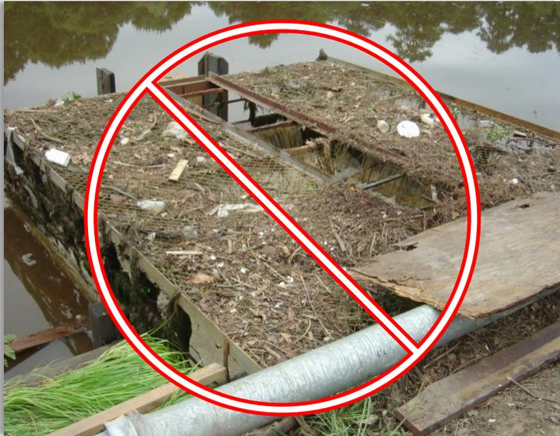
trash rack will allow debris to slide up to a higher elevation on the rack during high flow events without significantly impacting spillway capacity. For further guidance or assistance with specific trash rack applications and design references, please consult with Bureau engineers.
