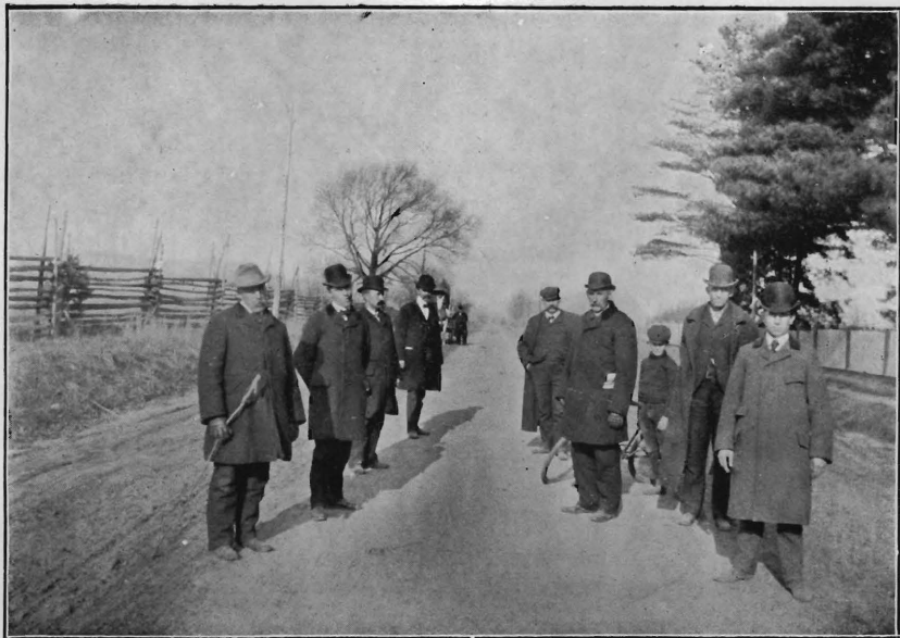
Jacksonville, Mt. Holly road, Burlington County, after improvement.
