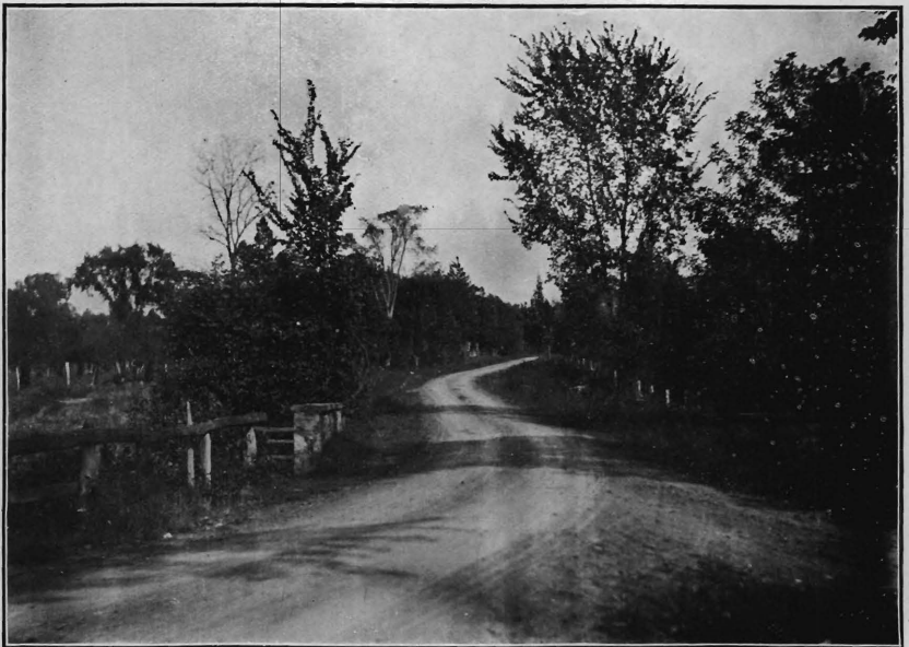
Eagle Rock Avenue, Essex County, after improvement. Eight-inch Telford.
