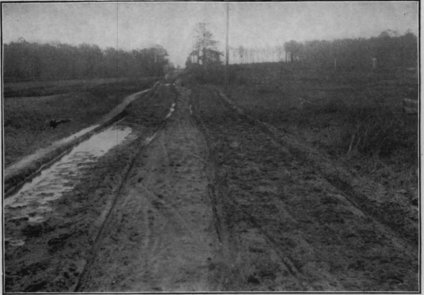
Seashore road, Cape May County, near Rio Grande, looking north, before improvement.
