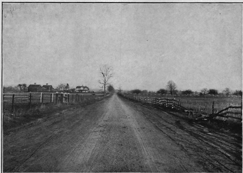
Bergen's Mill ore and stone road, Monmouth County. Four inches iron ore and four inches of trap rock.
