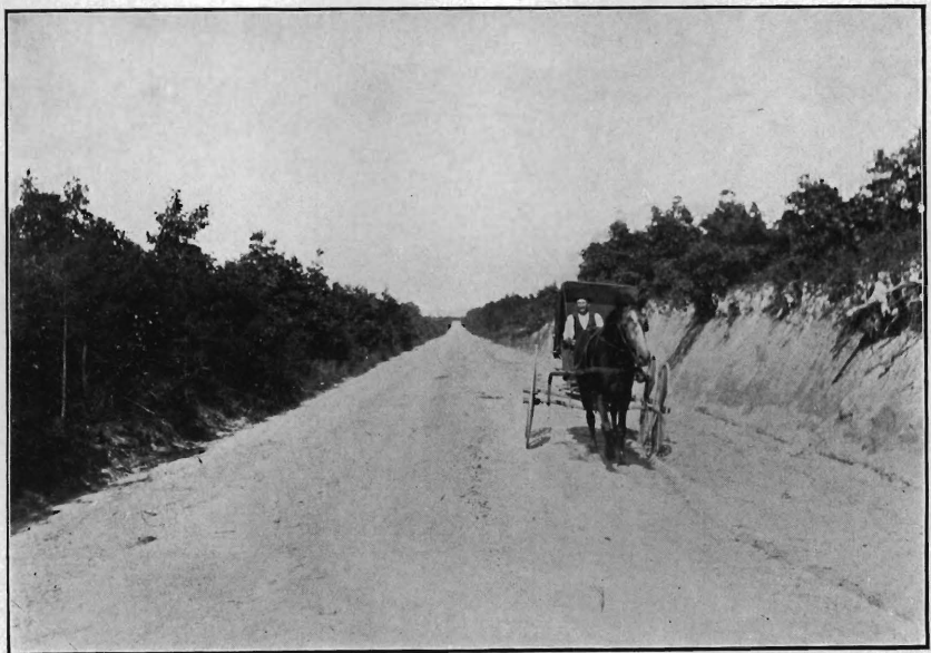
Egg Harbor and Greenbank road, Atlantic County, 1\frac{1}{2} miles out of Egg Harbor, showing cut after improvement.
