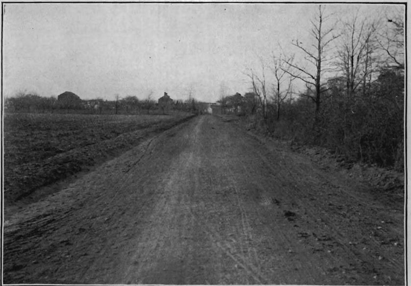
Key Port and Keansburgh road, Monmouth County, after improvement. Eight inch Macadam.
