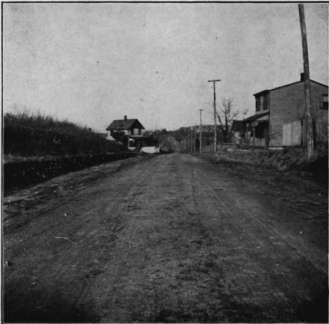
Haddonfield and Magnolia road, Snow Hill, Camden County, looking towards Haddonfield. Eight-inch Macadam.
