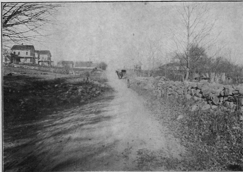
Echo Lake and West Milford road, near Baptist Church, Upper Macopin, Passaic County, looking north, before improvement.
