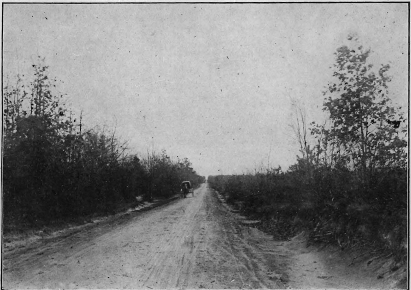
Stokes' Gravel road from Ballinger's Mills to Piper's Corner, Burlington County, after improvement.
