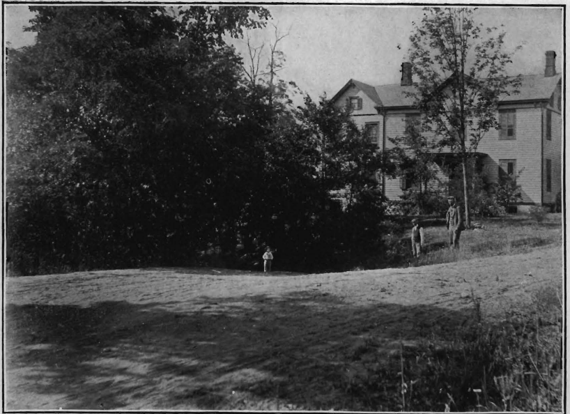
Pluckamin road at Moore's bridge, Somerset County, N. J., before improvement.
