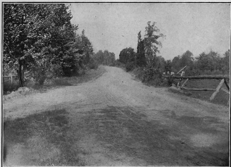
Eagle Rock Avenue, Essex County, before improvement.
