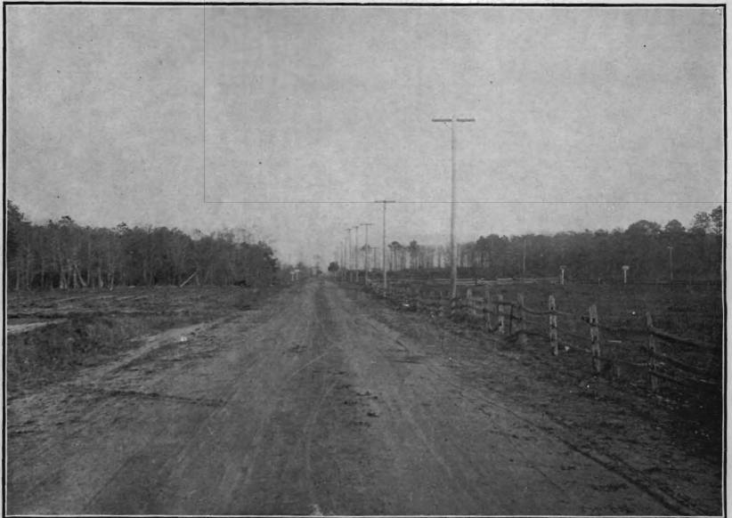
Seashore road, Gravel, Cape May County, near Rio Grande, looking north, after improvement.
