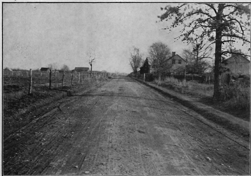
Key Port and Keansburgh stone road, Monmouth County. Eight-inch Macadam.
