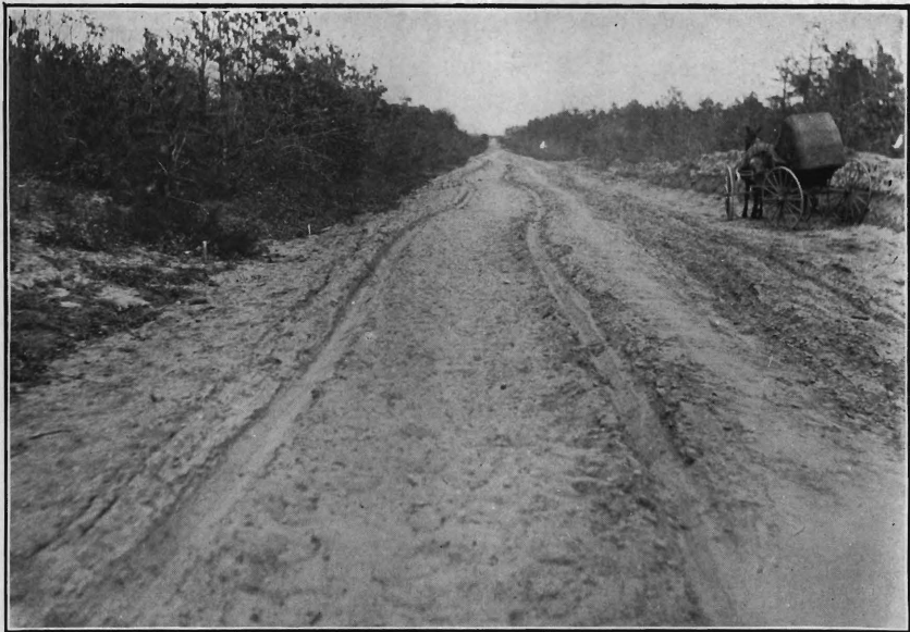
Egg Harbor and Greenbank road, Atlantic County, before improvement.
