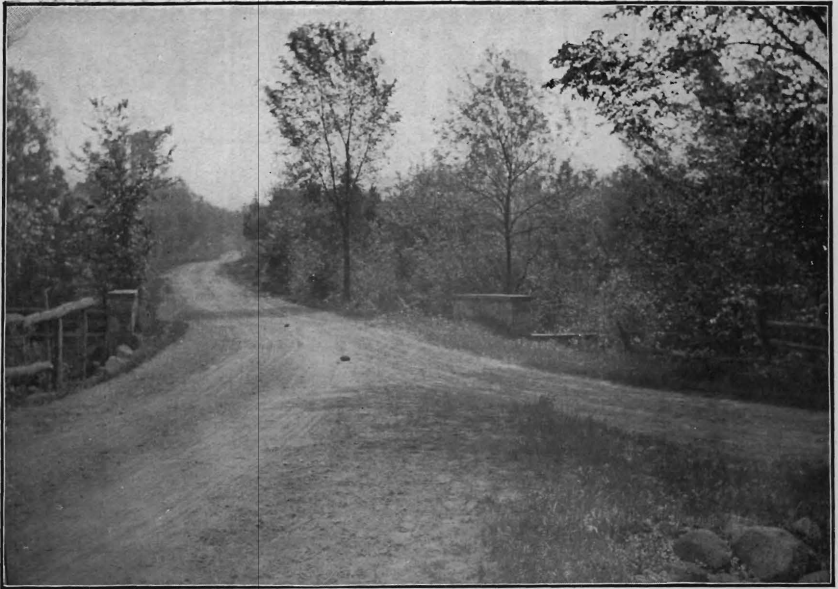
Eagle Rock Avenue, Essex County, before improvement.
