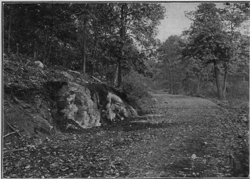
Cannon-ball road, Passaic County, after improvement, covered with fallen leaves. Four-inch Macadam.
