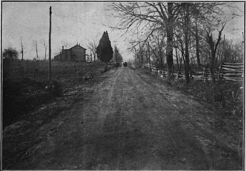
Hutton road, Burlington County, after improvement. Eight-inch Macadam.
