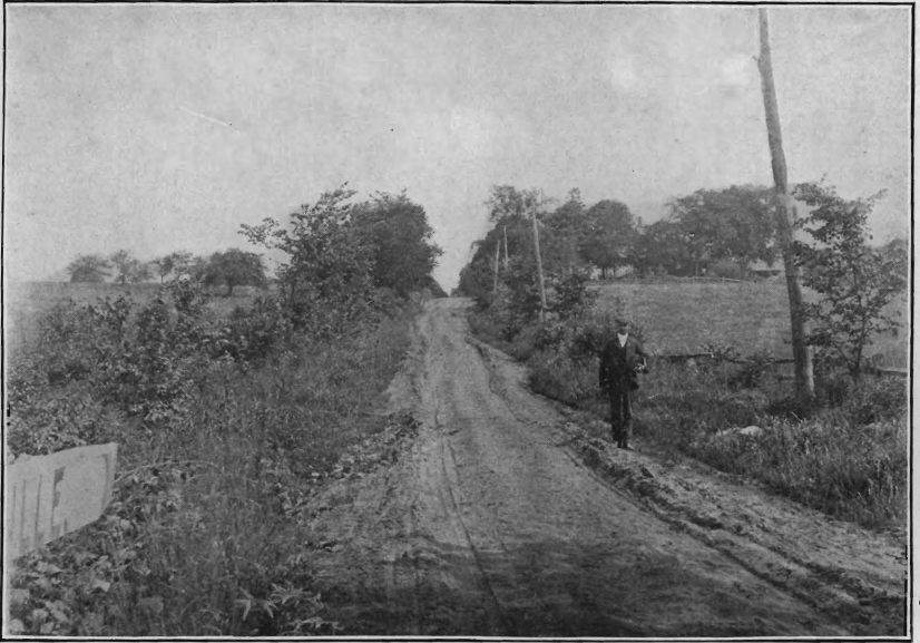
Pluckamin road, Hovey's Hill, Somerset County, N. J., before improvement.
