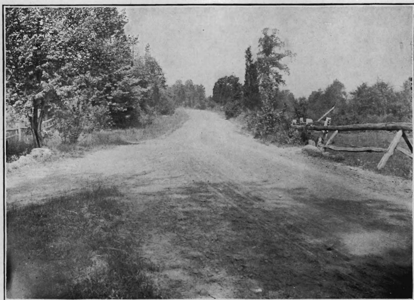
Eagle Rock Avenue, Essex County, after improvement. Eight-inch Telford.
