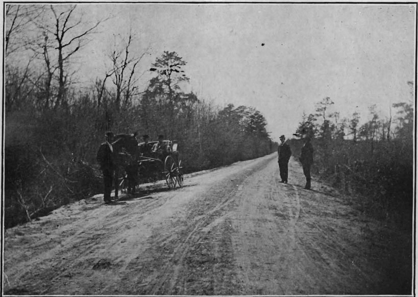
Wading River and Batsto gravel, Burlington County, through woodland and swamp, after improvement.
