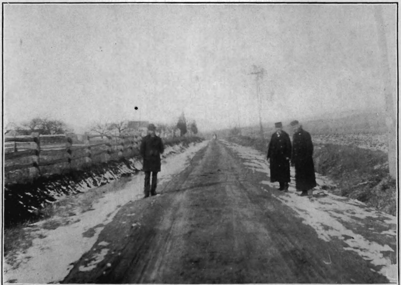
Pluckamin road, near Somerville, Somerset County, N. J., after improvement. Ten-inch rock bottom.
