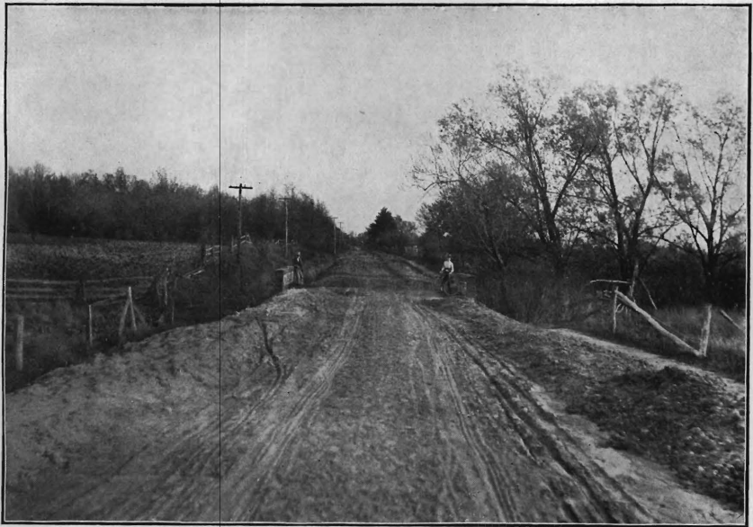
Cranbury and Hightstown road, Middlesex County, after grading.
