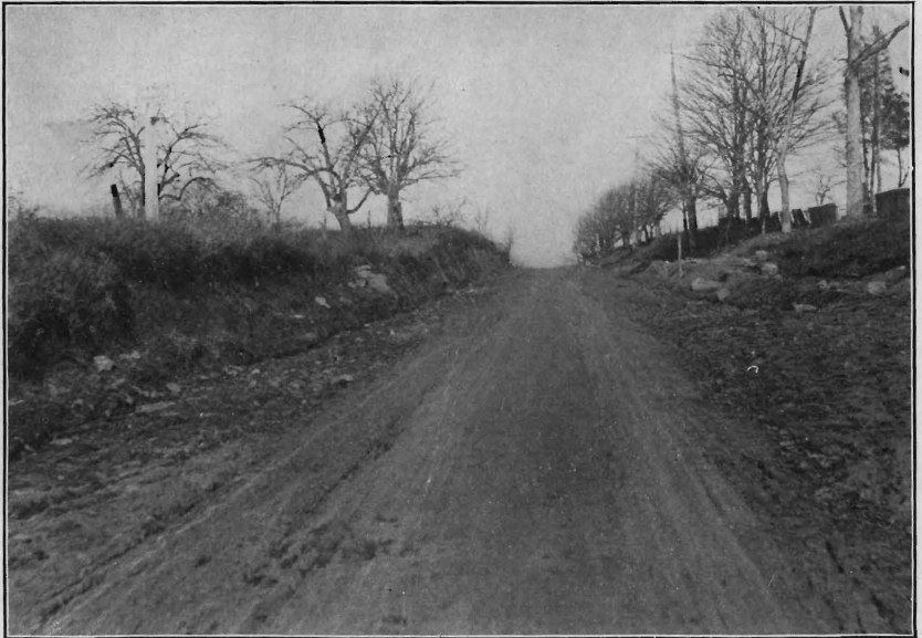
Pluckamin road, Somerset County, showing cut on Hovey's Hill.
