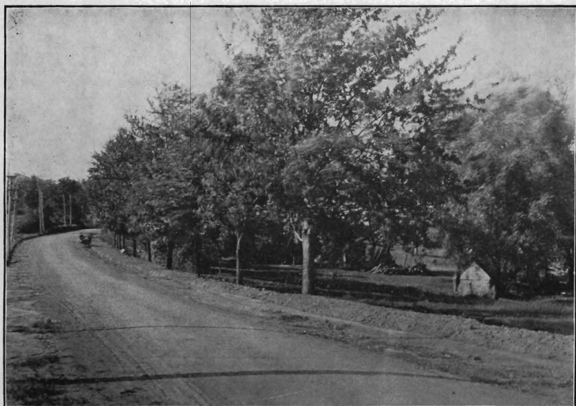
Kingsland Street, near railroad crossing, Franklin Township, Essex County, after improvement. Eight-inch Telford.
