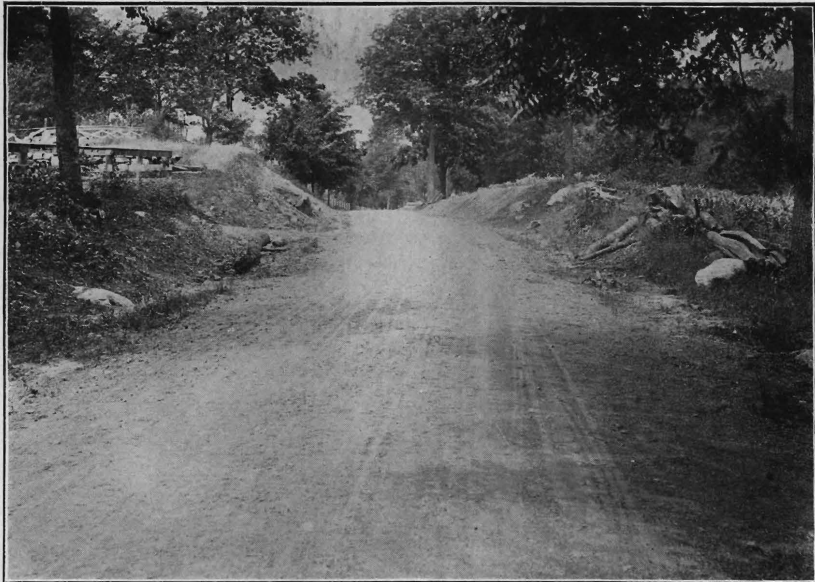
Echo Lake and West Milford road, Passaic County, northerly portion, after improvement. Four inch Macadam.
