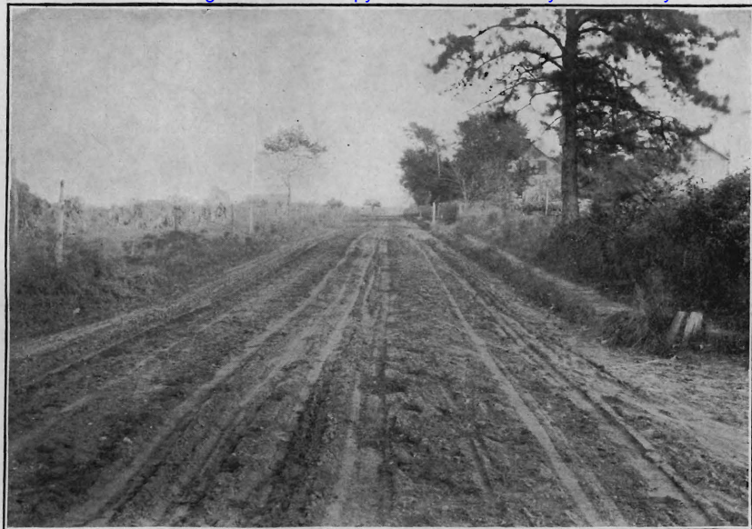
Key Port and Keansburgh road, Monmouth County, before stoning.
