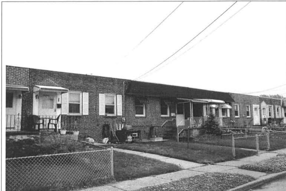
Photograph 2: 877-881 West Browning Road. Note the modern replacement doors and windows. View looking east (May 2004).
