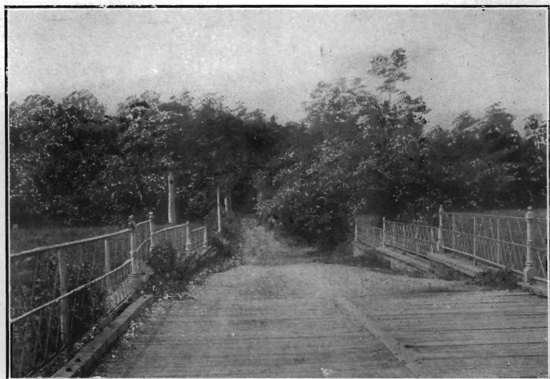
Princeton Hill Road, Mercer County Before Improvement
