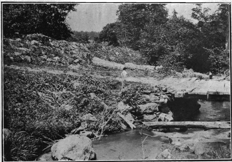
Tuttle's Corner Road, Sussex County Before Improvement
