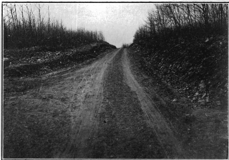
Mount Freedom Road, Morris County During Improvement.
