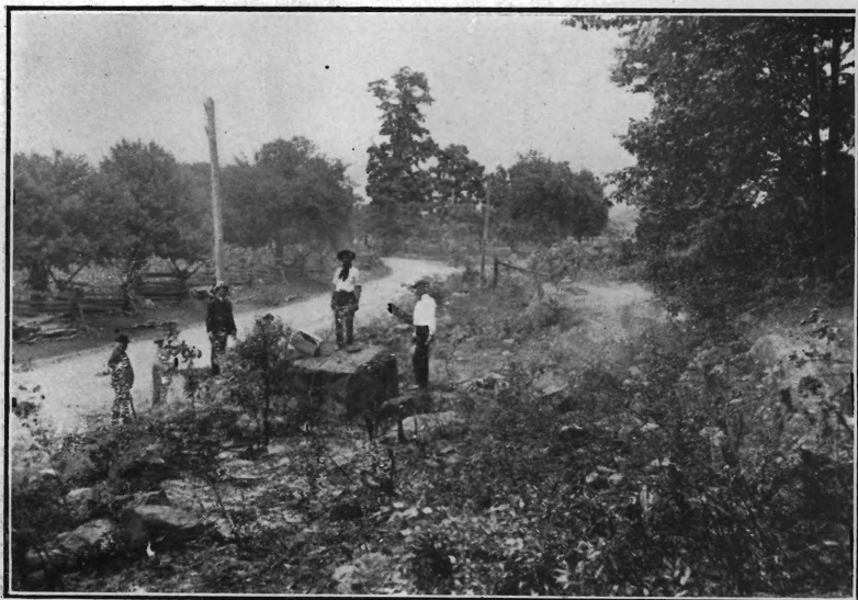
Roxburg Road, Warren County Before Improvement
