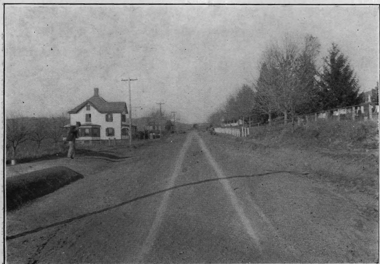
Peapack Road, Somerset County After Construction
