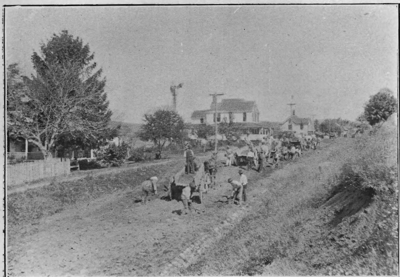
Peapack Road, Somerset County During Construction
