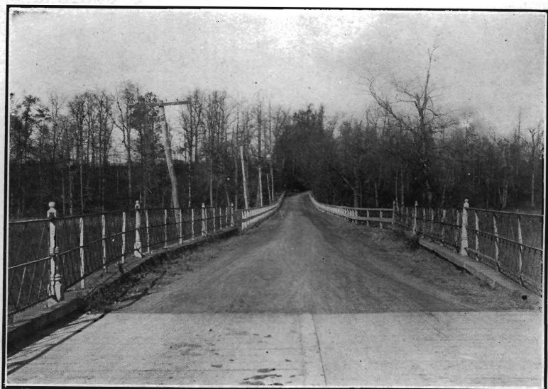
Princeton Hill Road, Mercer County After Improvement
