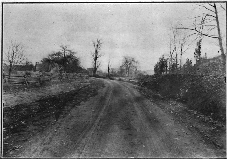
Roxburg Road, Warren County After Improvement
