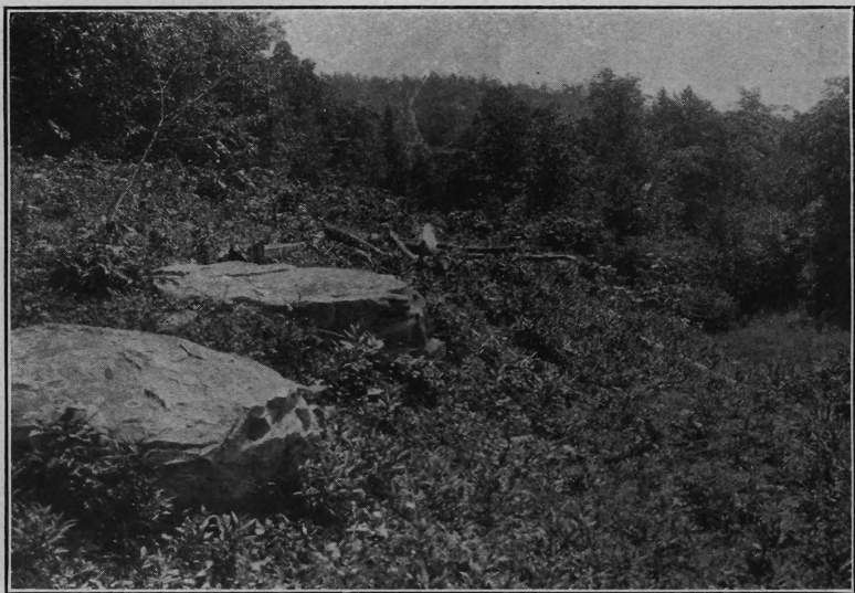
Tuttle's Cornor Road, Sussex County Before Improvement
