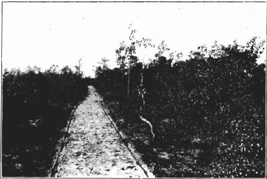
A woods road cleared out to serve as a fire line. Such a line, 15 feet wide, can be cut for $15 a mile.
