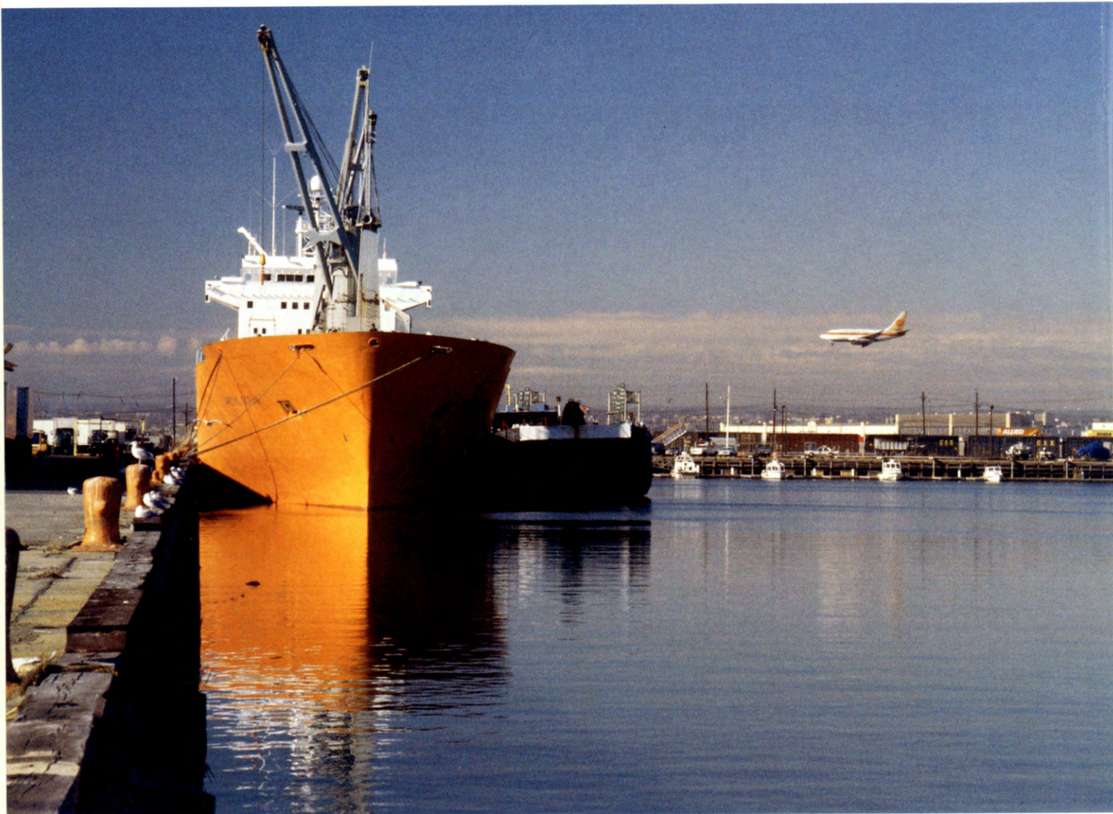
The Port Newark-Elizabeth Marine Terminal
