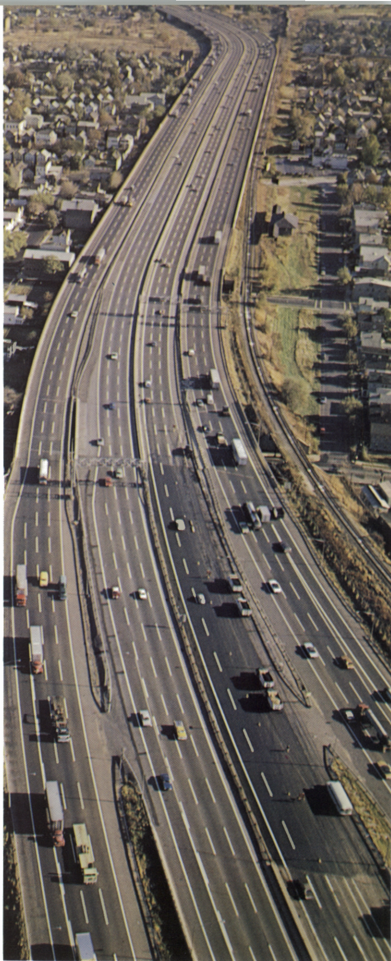
Traffic on the 12-lane dual/dual moves smoothly along the Turnpike at Elizabeth.
