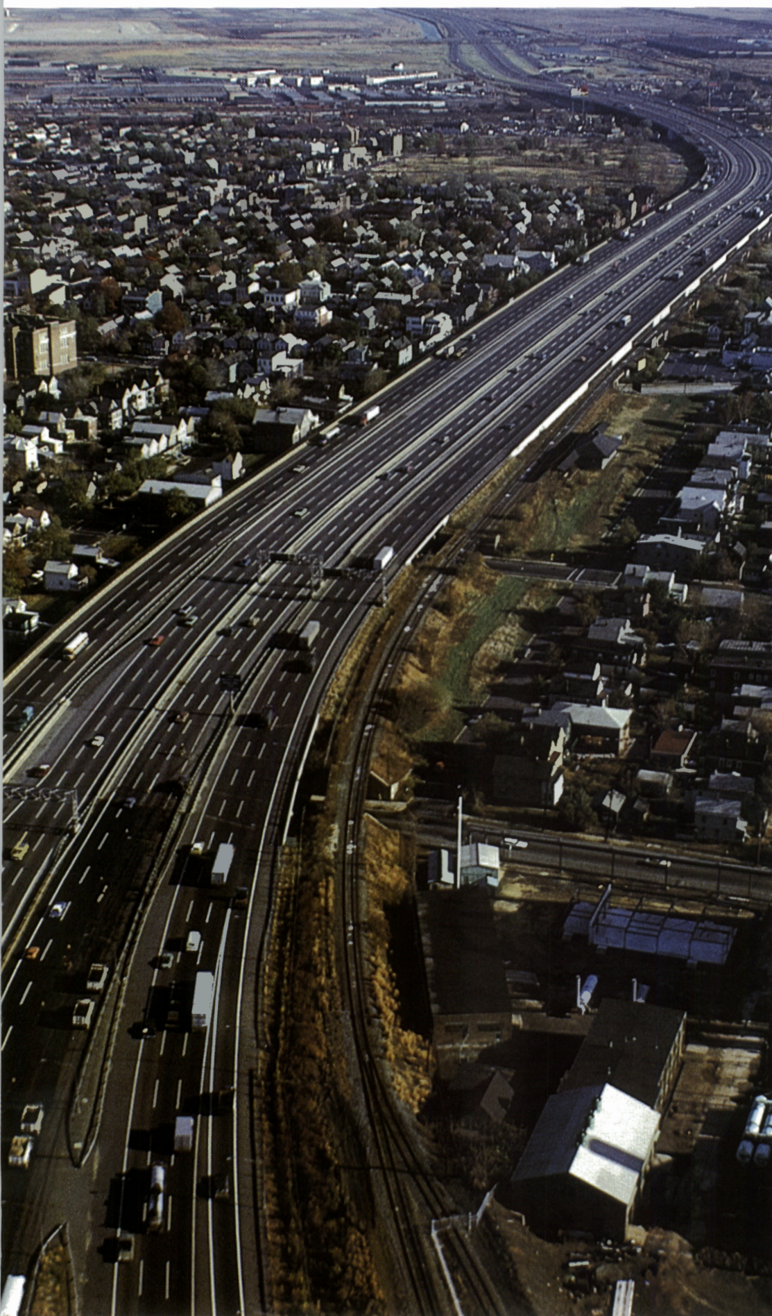
THE DUAL/DUAL: Twelve lanes, completed in 1970, custom-built to separate cars and trucks in innovative alignment.
