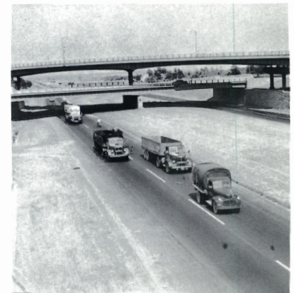
BACK IN THE '50'S: Four lanes in the Woodbridge area before the transformation...
