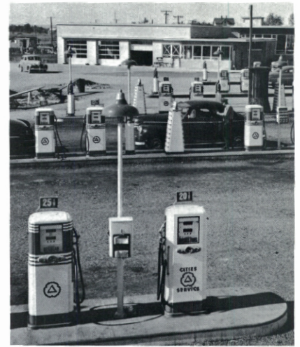
OLD SERVICE AREA: In place as Turnpike opened to traffic three decades ago.
