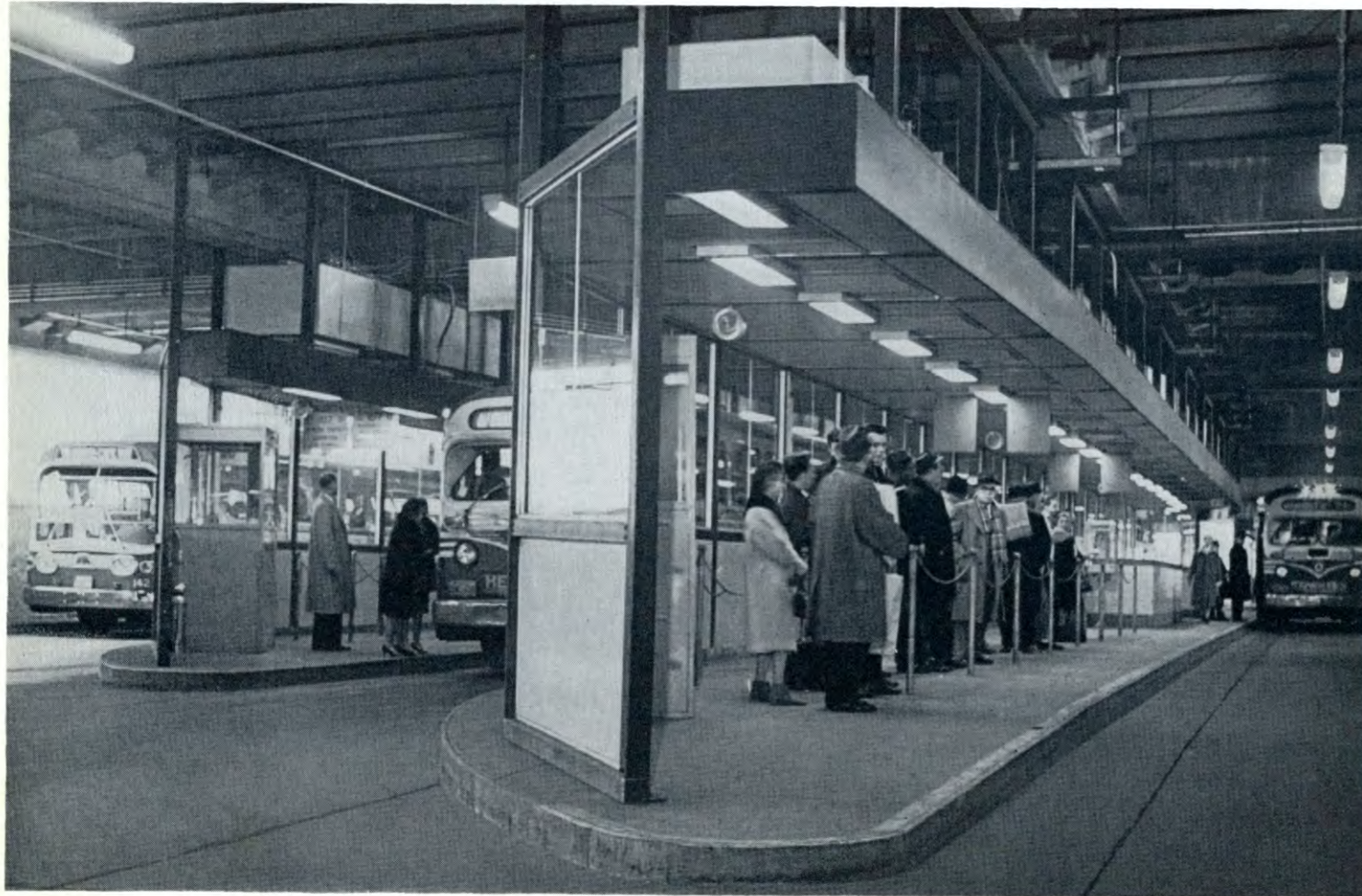
Three-sided glass enclosures provide protection against the weather on all of the Bus Terminal's suburban bus loading platforms.
