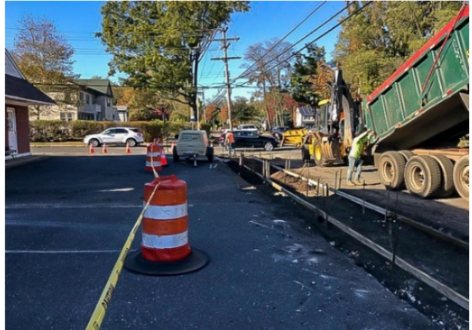
Borough of Little Silver - Sidewalk Project Phase II
