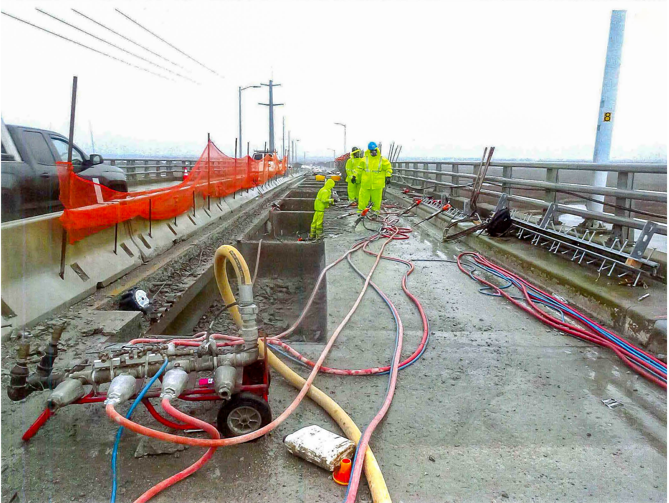
Cape May County – Avalon Boulevard (C.R. 601) over Ingrams Thoroughfare deck rehabilitation
