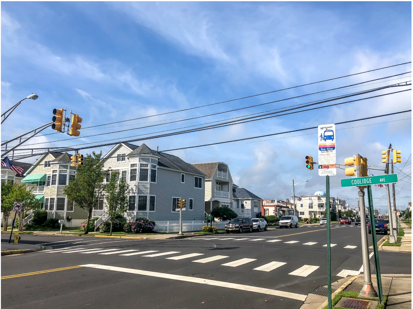
Atlantic County - Atl. Co. Rte. 629 Pedestrian & Traffic Signal Improvement Project
