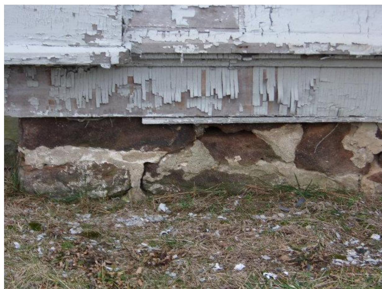
Stone foundation mortar repair
