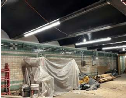
Platform LED light fixtures continue to be installed.
