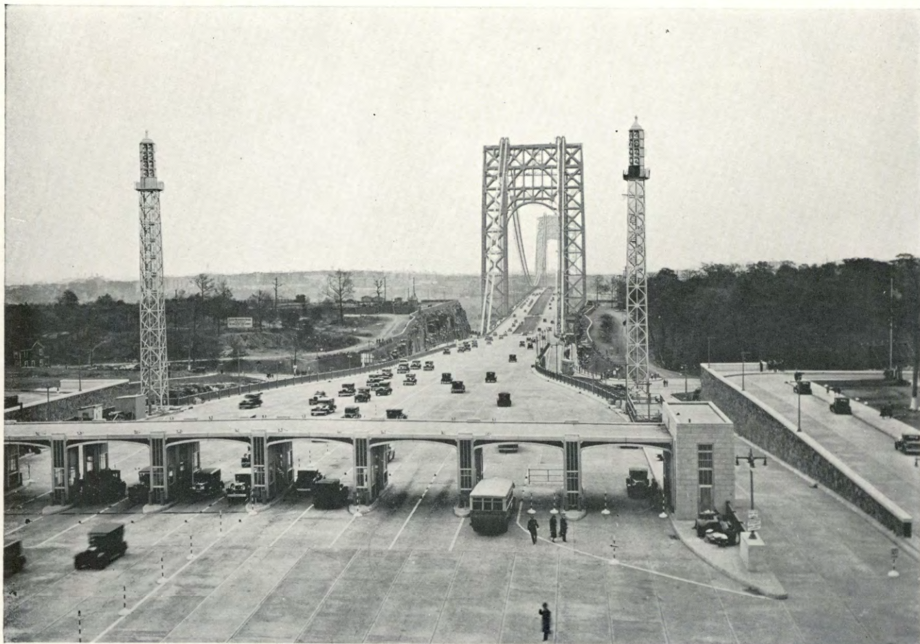
George Washington Bridge—Toll collection plaza on New Jersey Approach. November 1, 1931
