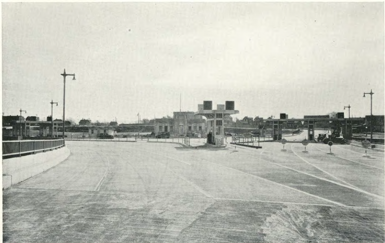
Bayonne Bridge—Toll Booths, Staten Island Plaza
