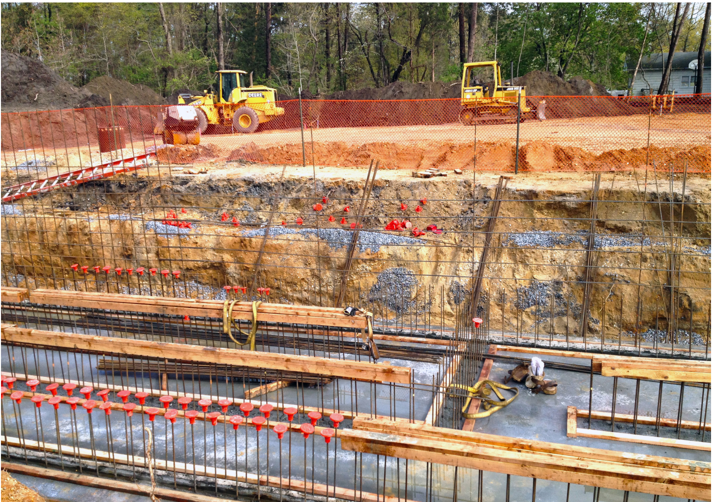
Millville City | Geissing Well No. 18 Concrete Clearwell Pit Foundation - SFY2013 Loan: $3,660,000
