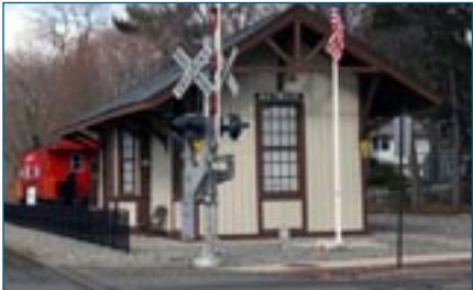
Maywood Train Station Restoration
