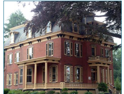
The John Hopkins House at 10 W. Main Street in Moorestown has been fully rehabilitated to serve as a real estate office.
