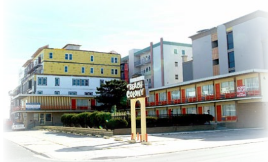
Beach Colony Motel in foreground and condominium construction in background
