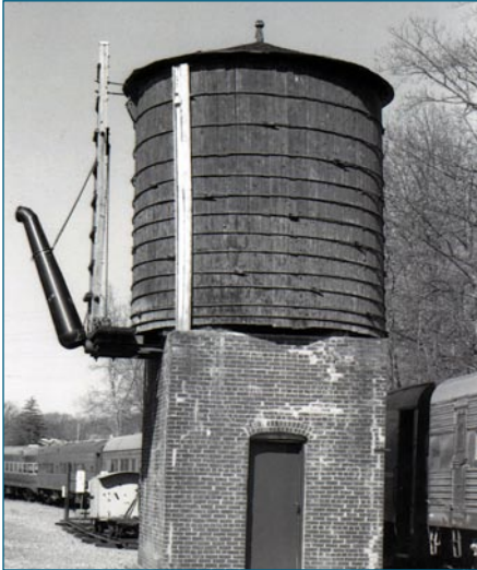
Morristown & Erie Railroad Whippany Water Tank
