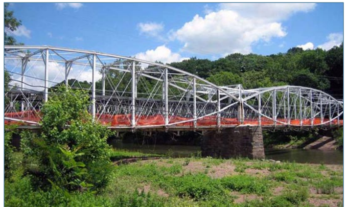
Elm Street Lenticular Truss Bridge
