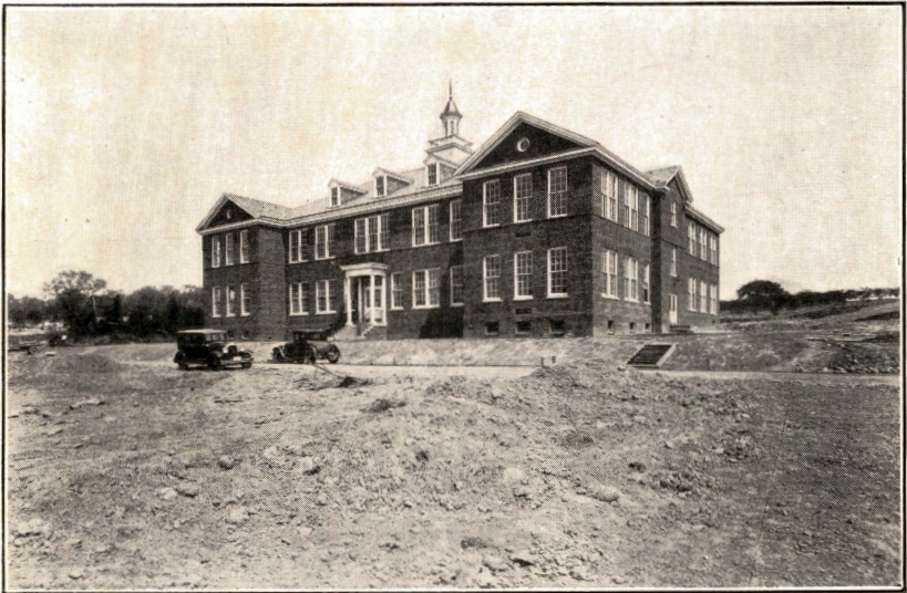
The School Building Nearing Completion
