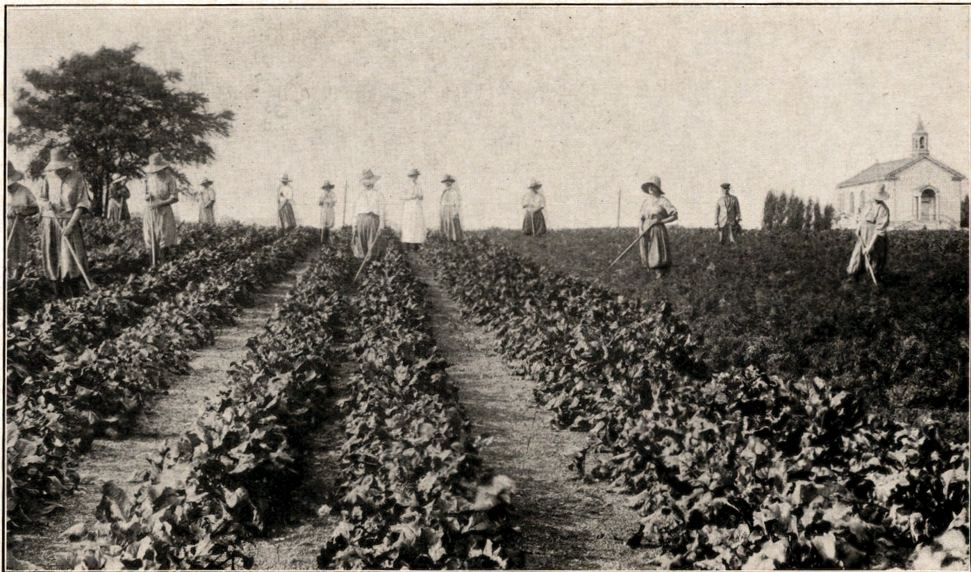
Wittpenn Chapel at Clinton Farms Reformatory
