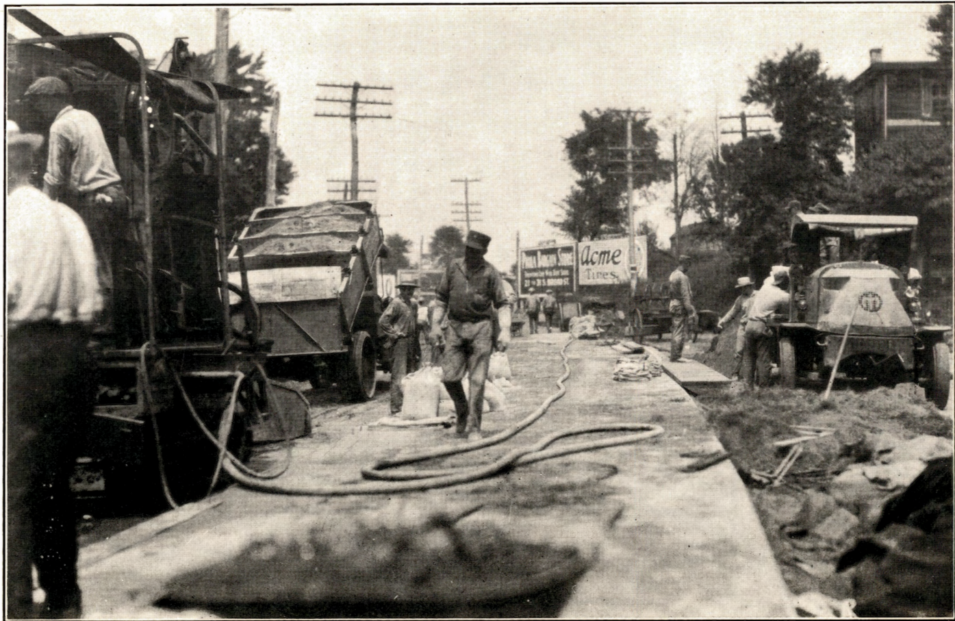
State Highway Construction by Prison Labor
