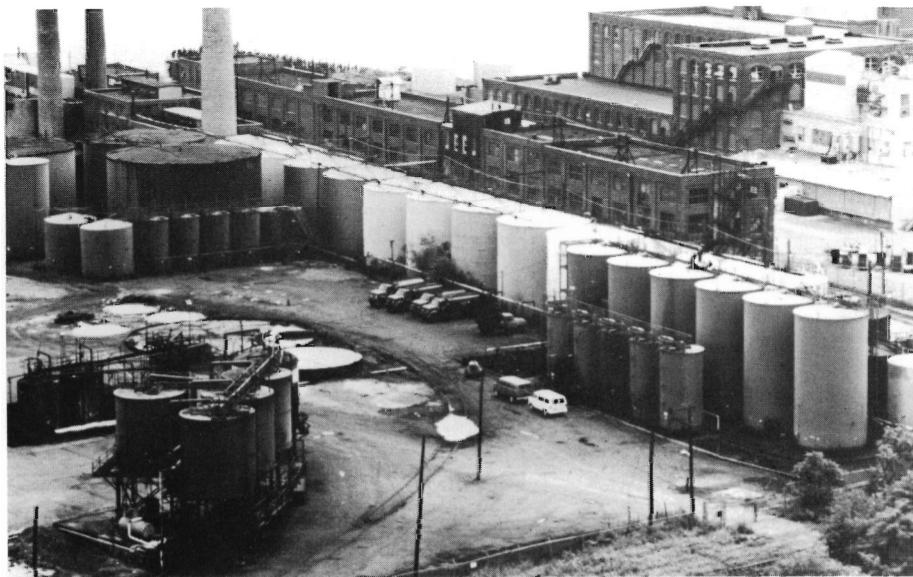
An oil recycling operation found illegally mixing hazardous wastes into its product. DEP Photo
