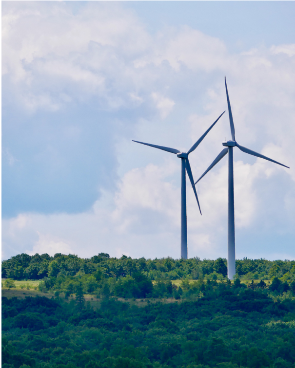
Casselman Wind Power Project in Pennsylvania.
