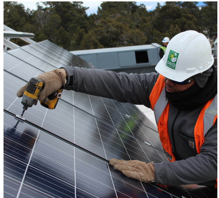
Installation of the San Miguel community solar array in Norwood, Colorado.
