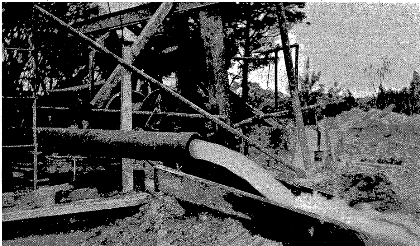
Discharge of new well at Margate City Water Works during preliminary test June 19, 1924. Rate of discharge 700 gallons a minute.
