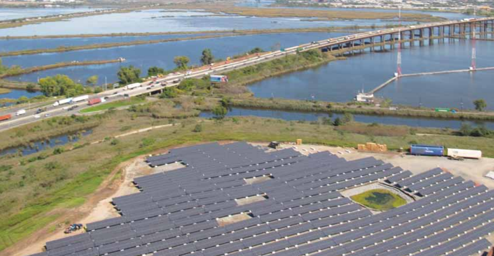
NJMC 1A Landfill Solar Project, Kearny
