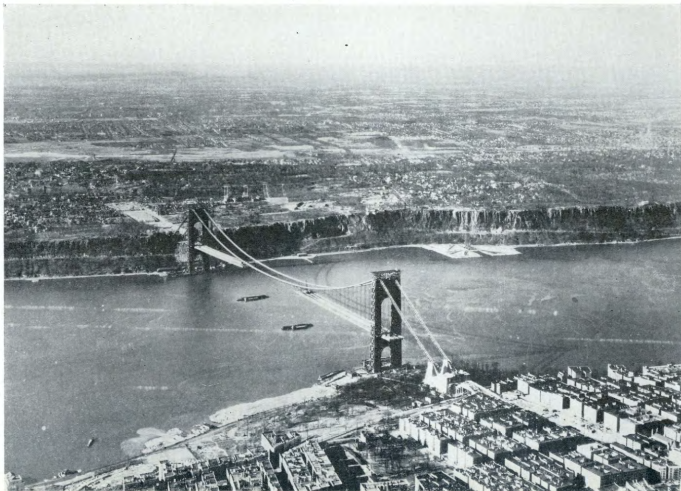
HR-1281—Aerial View of Hudson River Bridge Showing Status of Construction on December 13, 1930
