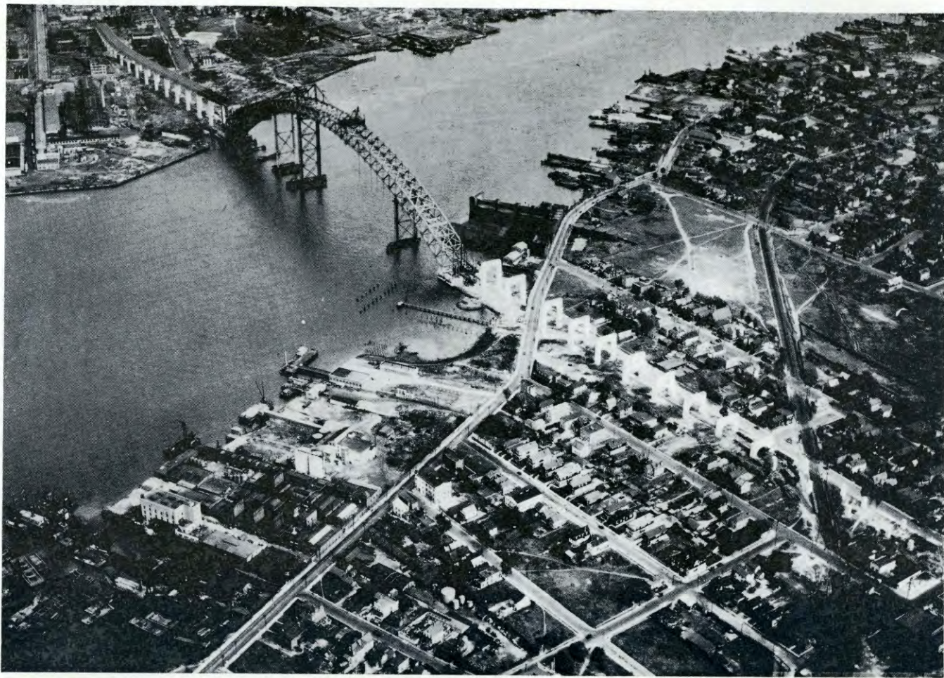
BP-586—Aerial View of Kill Van Kull Bridge. Port Richmond Approach in the Foreground. View Taken Following Joining of the Two Arch Sections on October 4, 1930
