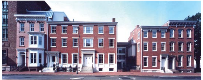
Exterior View of Townhouses after renovation and addition, DF Gibson Architects, PC Architect of Record
