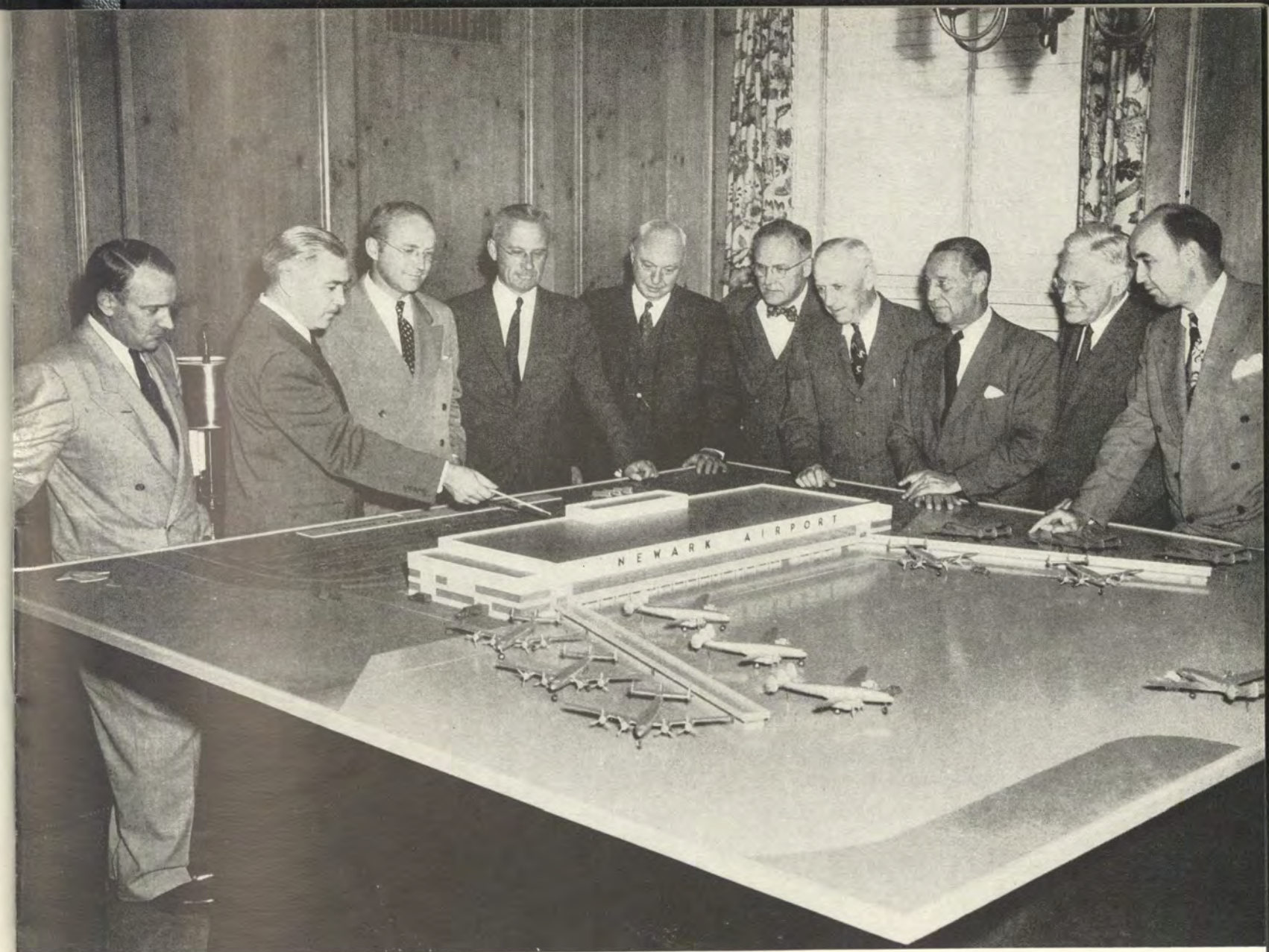
Executive Director Tobin discusses plans for new terminal building at Newark Airport as Commissioners and members of staff view model. Left to right, Chief Engineer Kyle, Mr. Tobin, Port Authority Commissioners Hamilton, Colt, Pope, Lowe, Armstrong, Chairman Cullman, Commissioner Corbin, and Director of Airport Development Glass.
