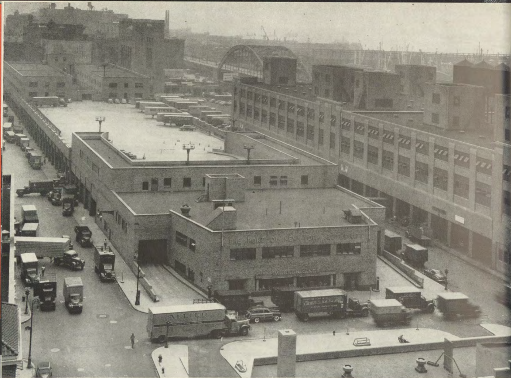
New York Union Motor Truck Terminal, spreading over four city blocks, is interchange point for less-truckload freight moving between metropolitan New York area and points throughout the country and overseas. Outgoing freight picked up by fleet of local trucks is consolidated into truckloads at the terminal; local trucks also deliver to consignees freight assorted from loads on incoming over-the-road trucks.
