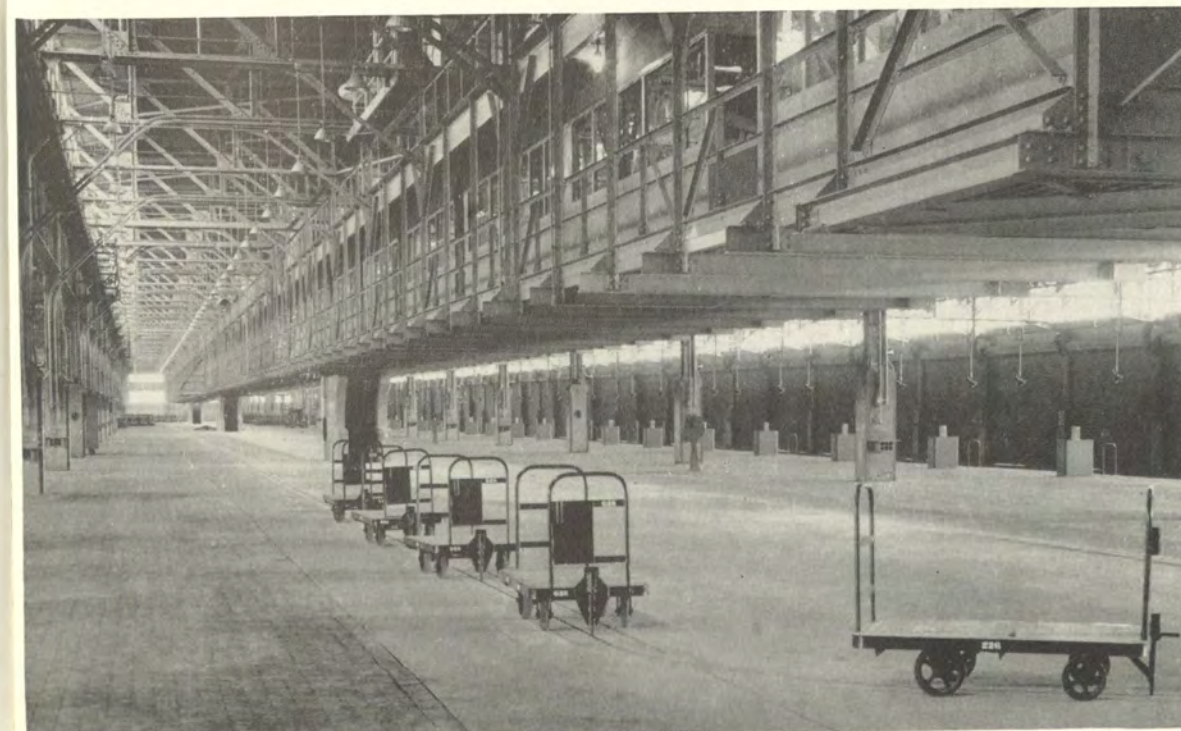
Interior of Newark Union Motor Truck Terminal, photographed on its completion. Endless conveyor for moving freight differs from New York Union Motor Truck Terminal in having its mechanism under floor instead of overhead.
