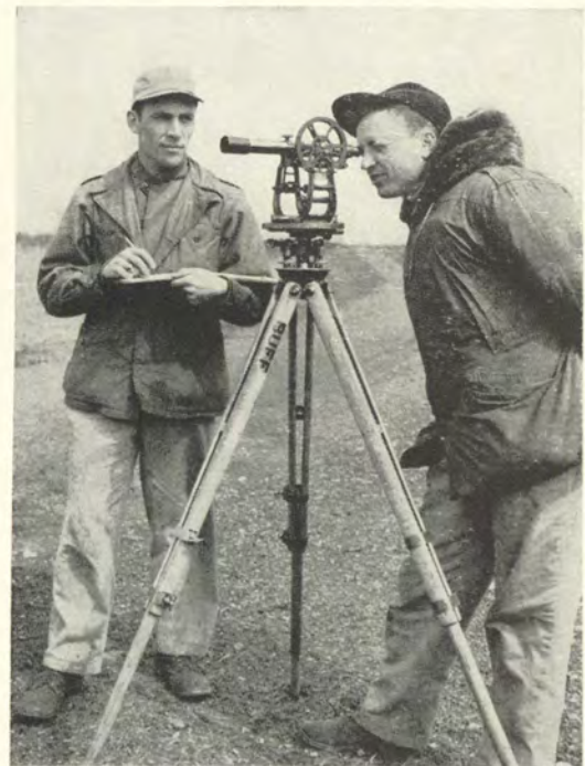
Chief of field survey party, John M. Kaelberer, takes notes on reading by Engineer Robert Shepard in survey for fill at Newark Airport.
