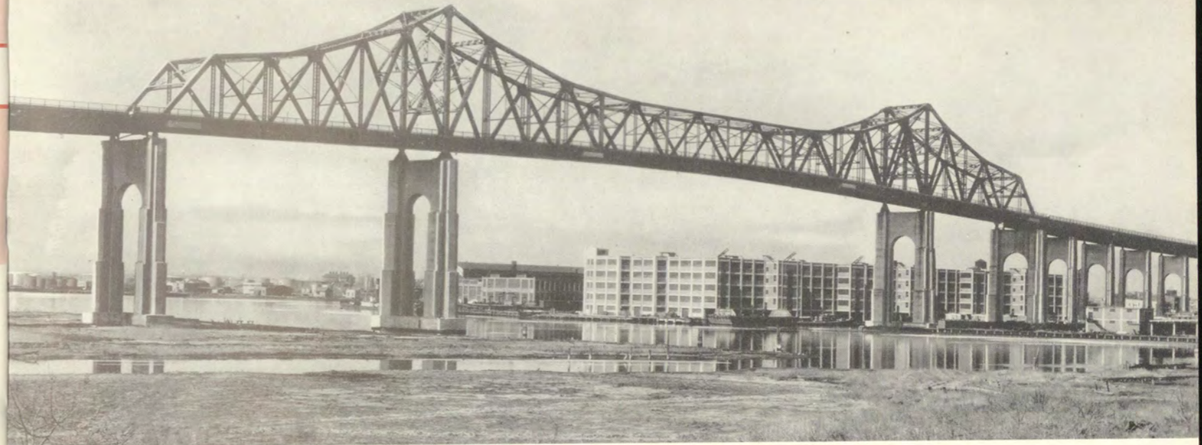
1928—GOETHALS BRIDGE (above) and OUTERBRIDGE CROSSING (below). These great cantilever bridges over the Arthur Kill join Staten Island with Elizabeth and Perth Amboy, New Jersey. The first two of the Port Authority's sixteen transportation and terminal facilities were built at a cost of $17,000,000. They were named for General George W. Goethals of Panama Canal fame, the Authority's first consulting engineer, and for Eugenius H. Outerbridge, its first chairman.
