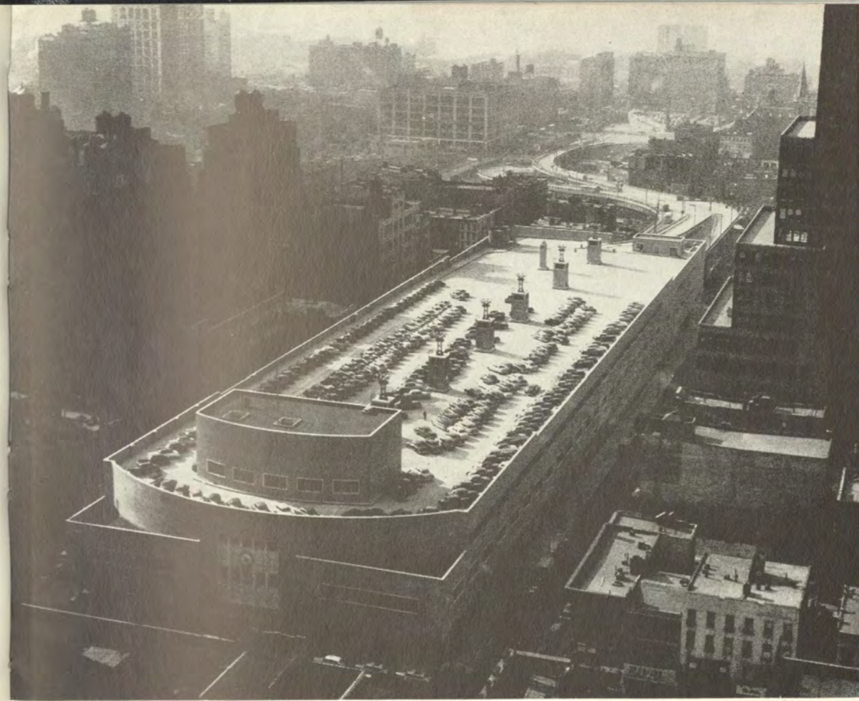
The Port Authority Bus Terminal showing main entrance, roof parking area, and ramp to Lincoln Tunnel.
