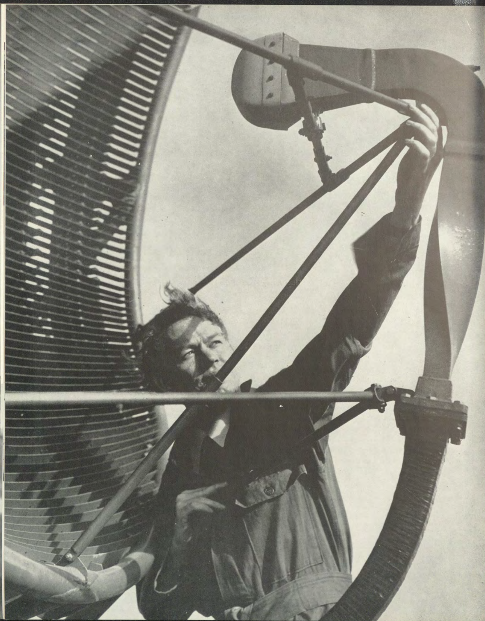
Technician making adjustments to airport surveillance radar equipment which indicates location of aircraft within a range of 30 miles of La Guardia Airport.
