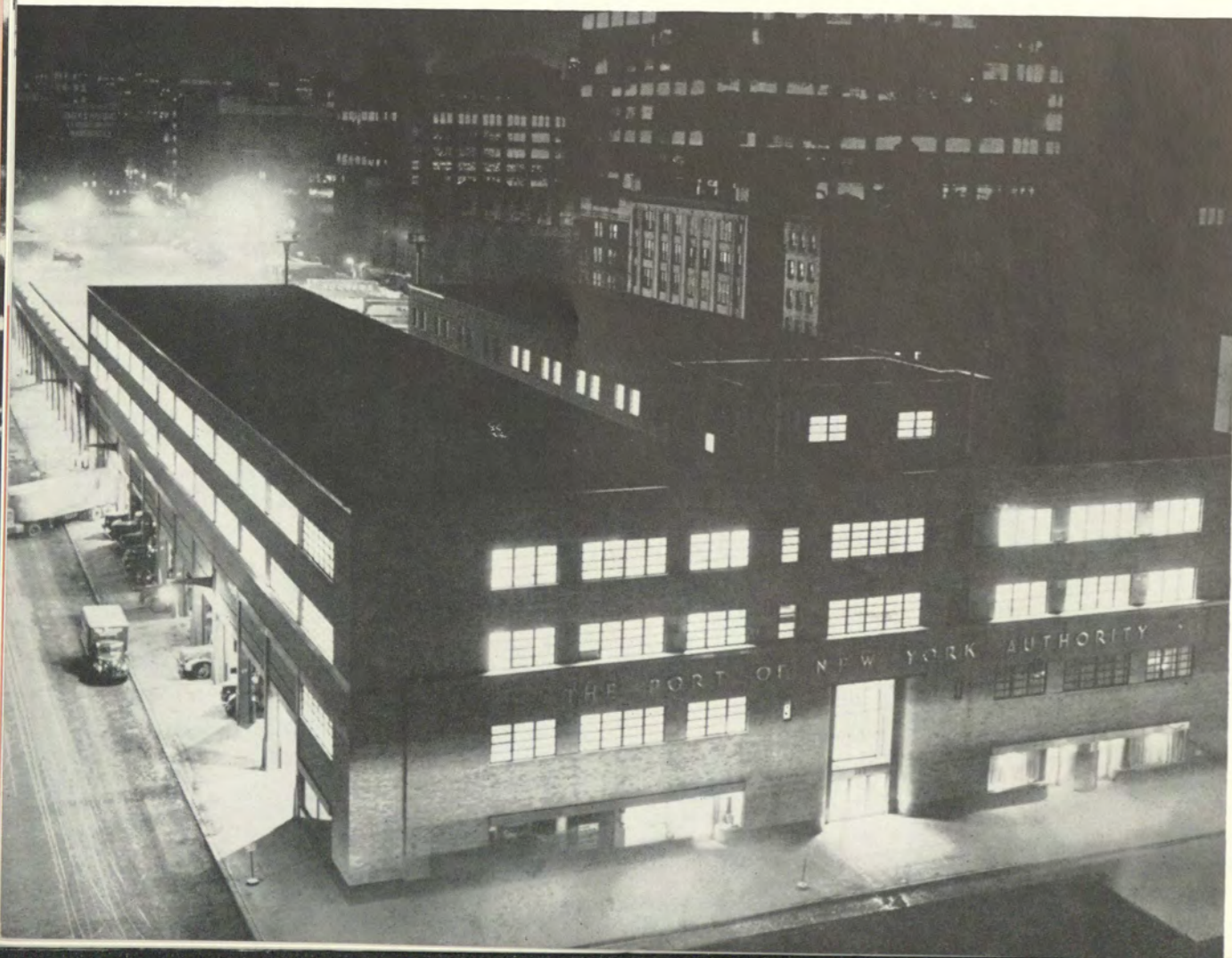
1949—NEW YORK UNION MOTOR TRUCK TERMINAL. The first of two such terminals built by the Port Authority in the New Jersey-New York Port District, it occupies four blocks in lower Manhattan near the Holland Tunnel and the Hudson River steamship piers. The $10,000,000 terminal is designed to reduce street congestion and handling costs and to provide modern facilities and equipment for the transfer of truck freight. All trucks park in bays off street.
