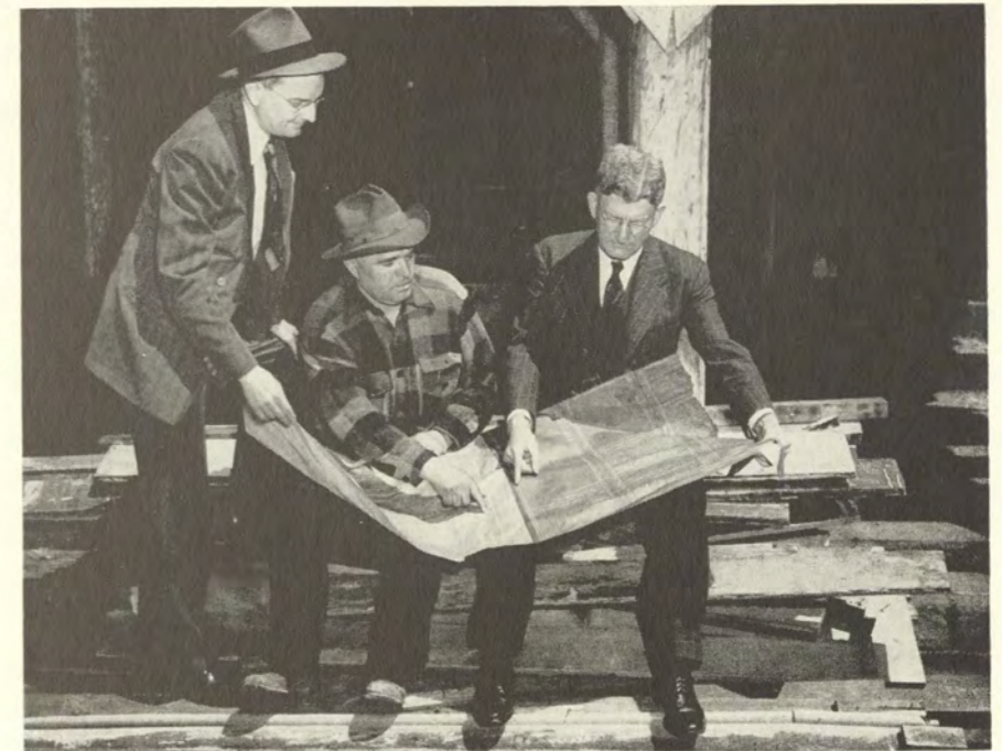
Before Bus Terminal construction began Lee C. Webb, Superintendent of the Bus Terminal (left), discussed plans with George Cosman, Supervisor of Demolition, and Harvey S. Quigel, Port Authority Director of Real Estate.
