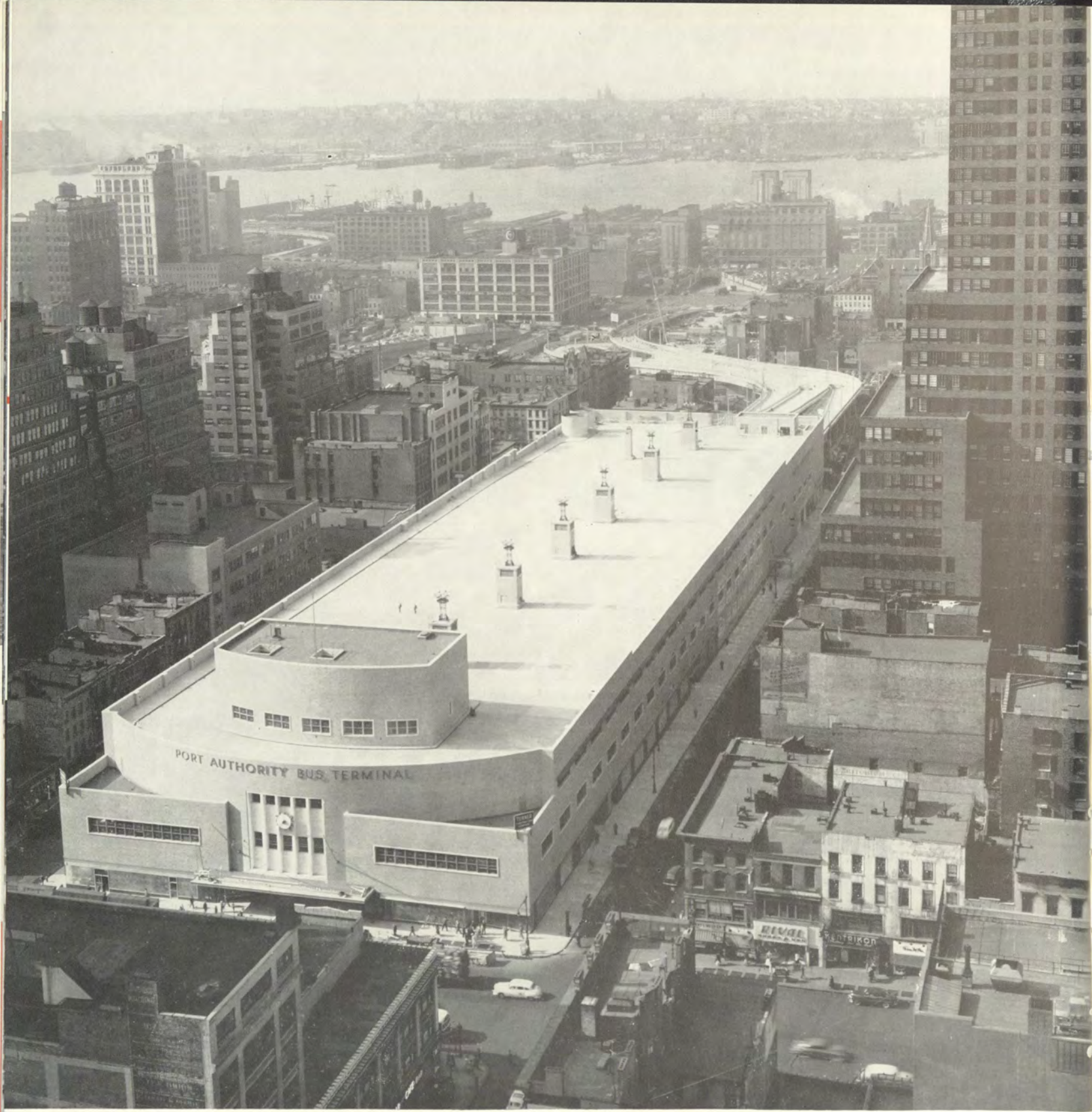
1950—PORT AUTHORITY BUS TERMINAL. One block from Times Square, this huge terminal, largest in the world, serves more than 130,000 long distance and commuter bus passengers. At the same time, by means of direct ramp connections with the Lincoln Tunnel, the $24,000,000 structure relieves the crowded Manhattan streets of about 85 per cent of the 2,500 interstate buses which enter midtown daily.
