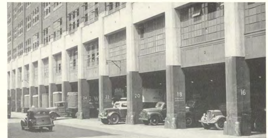
Close-up of off-the-street truck bays on the 15th Street side of the Union Railroad Freight Terminal, in Port Authority Building, for consolidation of less-carload rail freight.
