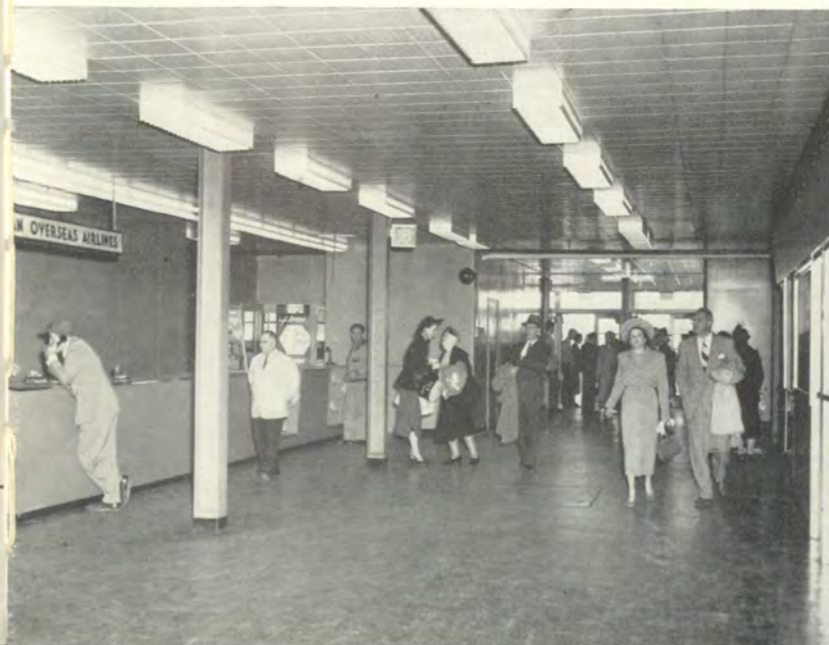
International travelers in the new two-story addition to the Terminal Building.
