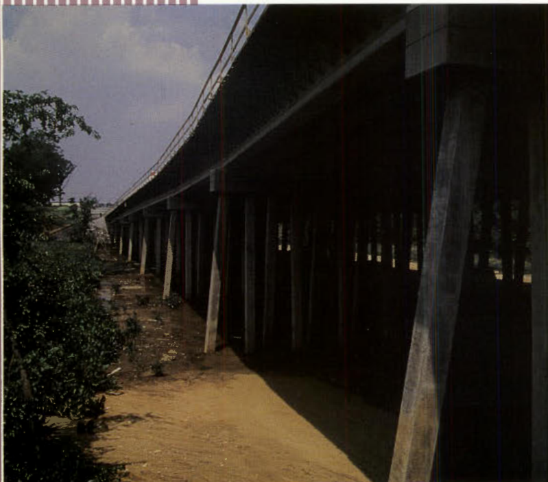
Route 70 Bridge over Bear Swamp Road
