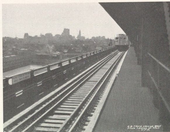
TRANSIT LINE ON BRIDGE
