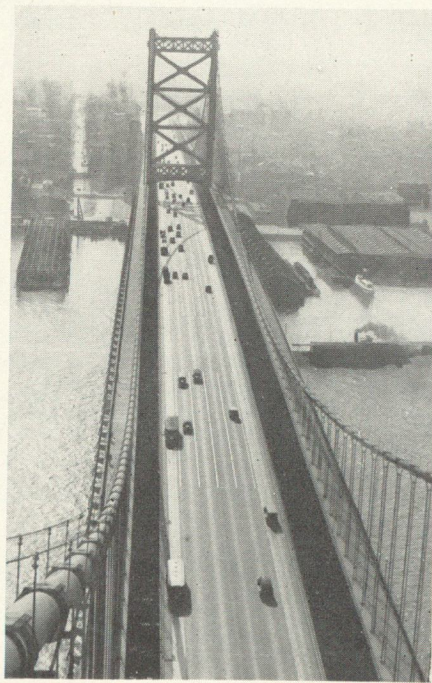
DELAWARE RIVER BRIDGE FROM TOP OF TOWER
