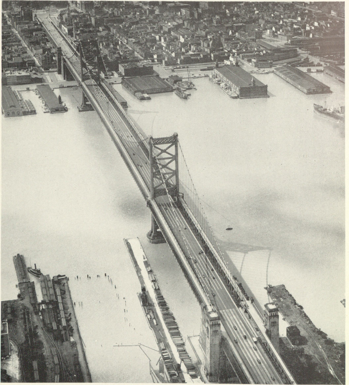
DELAWARE RIVER BRIDGE
