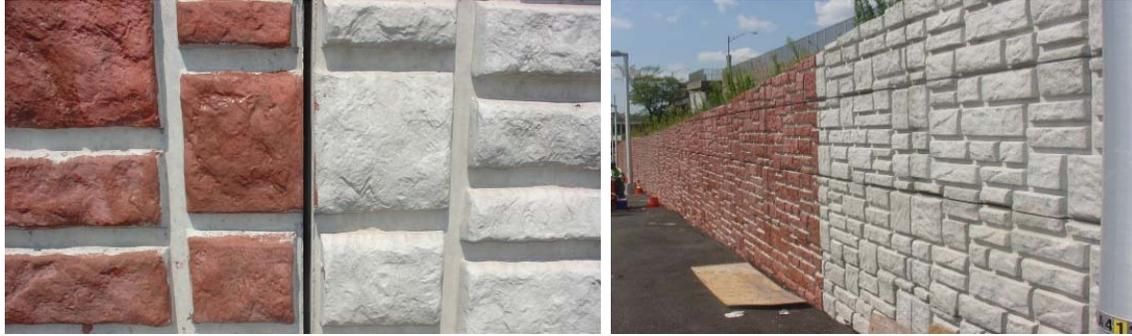
Figure 2. Contrast between Parent and Coated Surfaces
