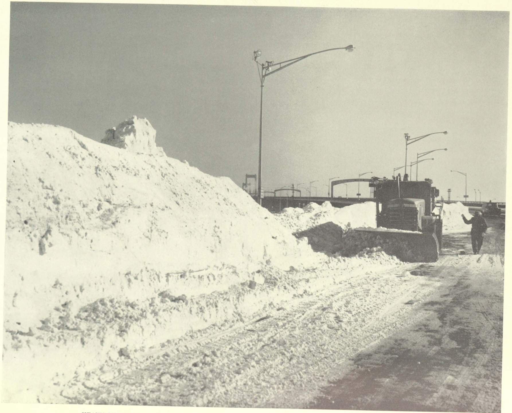
HEAVY SNOW FROM DECEMBER BLIZZARD IS CLEARED FROM ROADWAY AT WALT WHITMAN BRIDGE.
