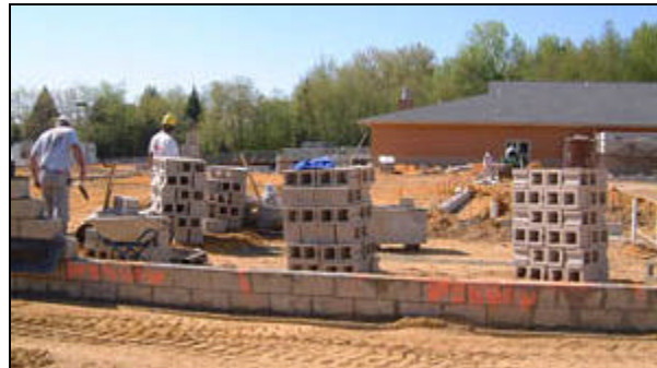
Work progressing on the Johnstone site
