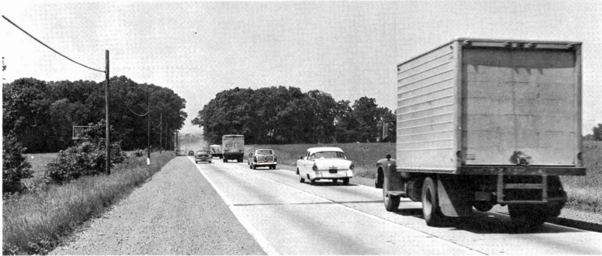
A major item in the determination of roadway adequacy is surface width. Determination of tolerable surface widths were based on requirements for traffic capacity and for traffic safety. Tolerable widths vary with a route's functional classification and traffic volume.
