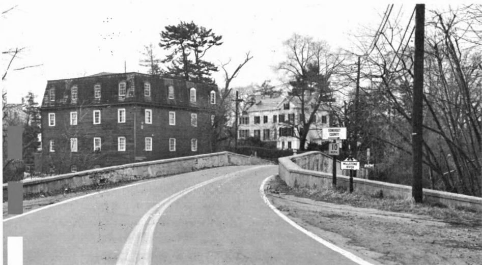
Roadway alignment was one of the items evaluated in the appraisal of needs as was structure width. Alignment is the major design element affecting operational characteristics of a facility and is, therefore, primarily related to functional classification or level of service. Structure width is a major item in the evaluation of highway safety because of the hazards imposed by narrow clearances to bridge abutments.
