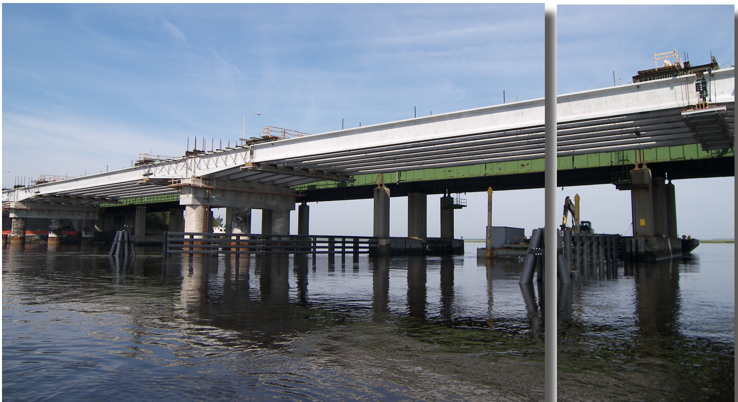
Parkway Widening - Mullica River Bridge
