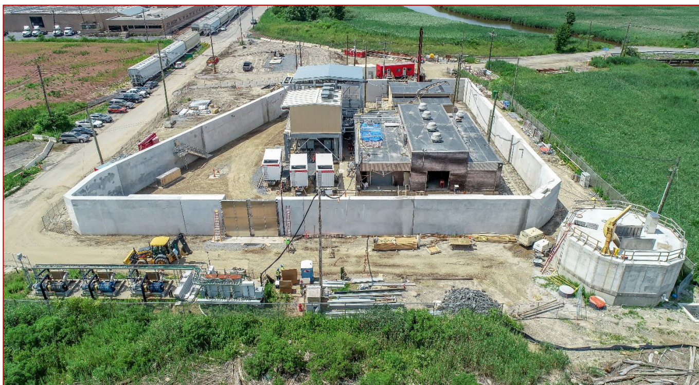
Restoration and Flood Mitigation
