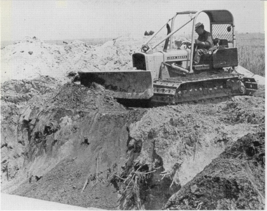
After proper leveling, the pipes are covered with fill
