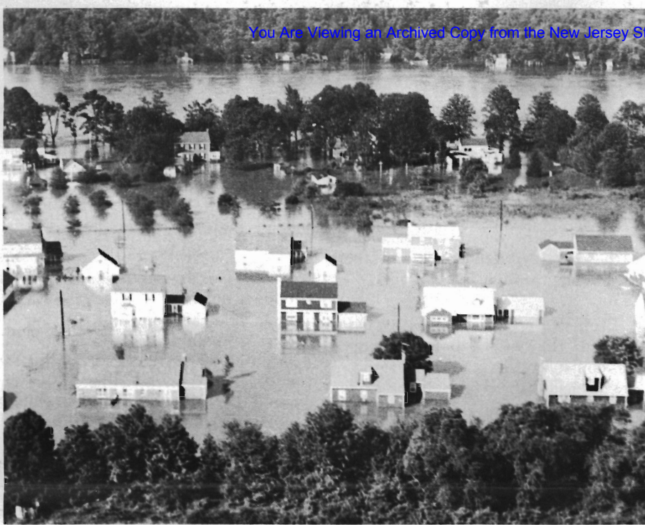
FLOOD —These relatively new homes in the Trenton area were inundated by the flooding Delaware River (background) in 1955. The Land Use Act would regulate the development that could occur on flood plains.
