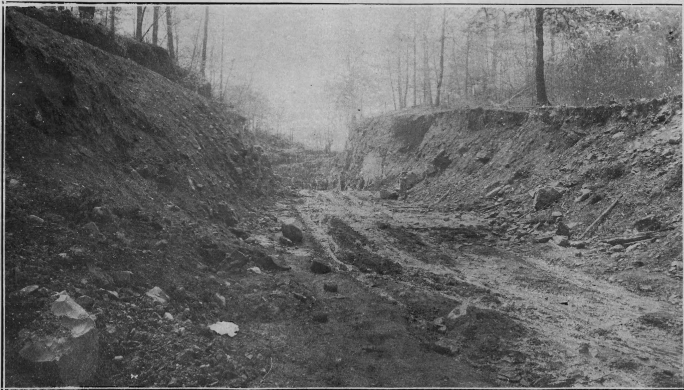
Showing how grade was reduced on Normal Avenue, Essex County.
