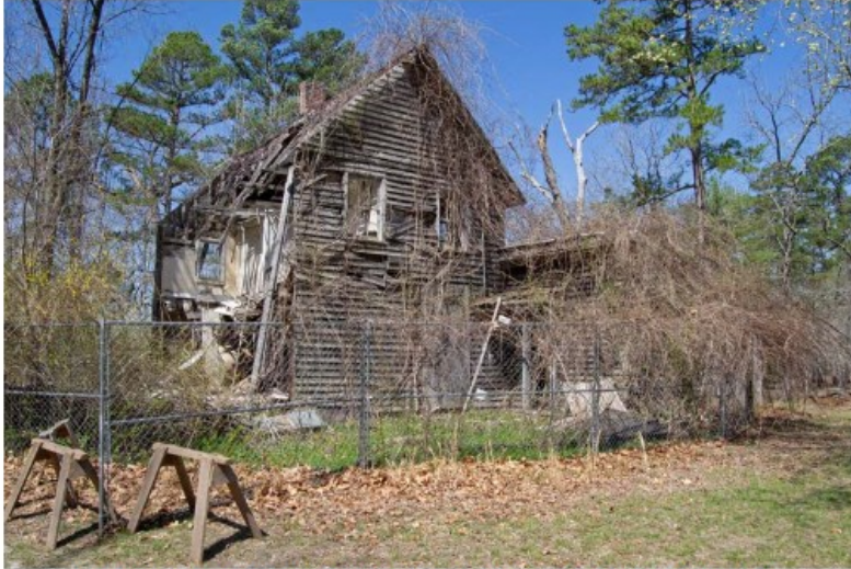
Photo 3: View of building from the southeast, April 10, 2025.
