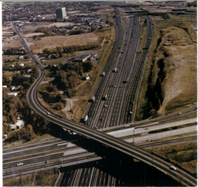
The Turnpike dual/dual at Woodbridge under the Garden State Parkway and Main Street bridge in X-formation.
