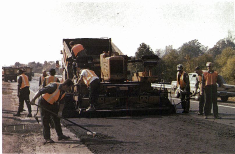
Maintenance crew resurfacing section of mainline.
