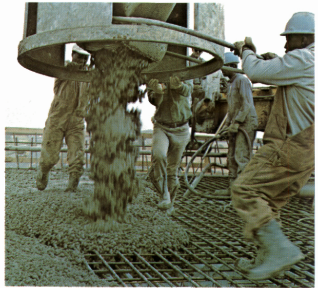
As at a town meeting, the good folk (left) gather at Manalapan High School for public hearing on Toms River Expressway on December 12. Workers (below) are pouring concrete over steel reinforcing rods for one of many bridge decks.
