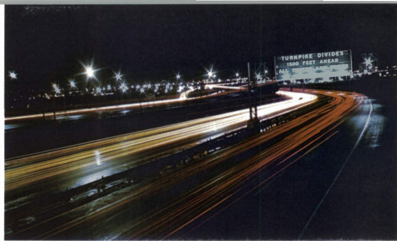
Night traffic light-streaks along the "mixing bowl" approaching the 12-lane section.
