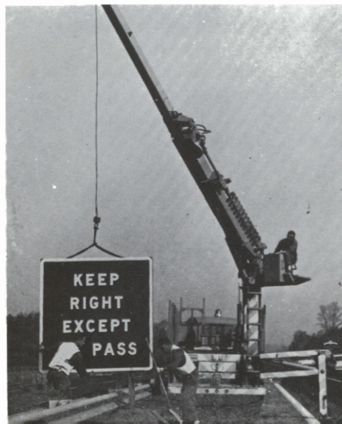
Newly - formed bridge painting operation at work on one of the numerous overpasses, using hydraulic lift truck. At left, truck boom being used to erect new, larger signs.
