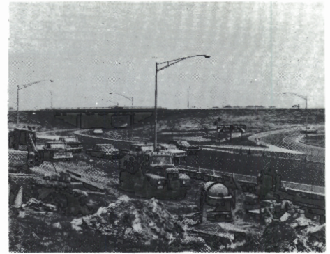
Additional exit lane under construction at Interchange 9, New Brunswick, by Turnpike Authority's maintenance men and equipment.
