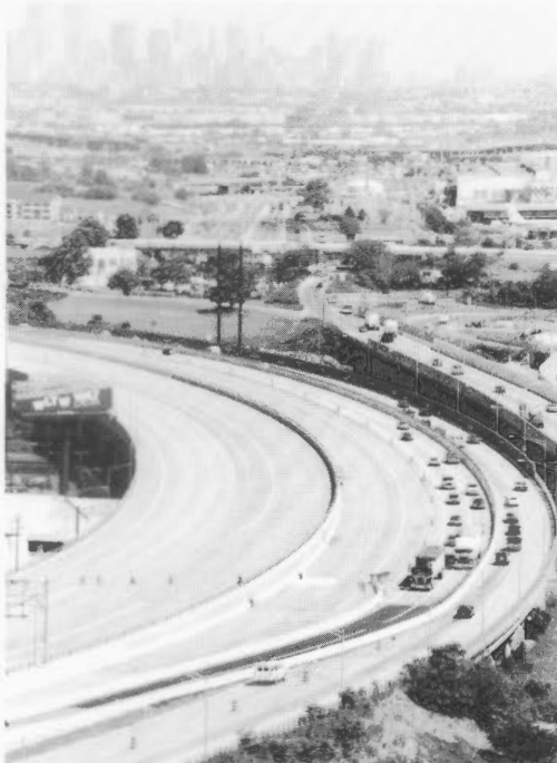
THE I-78 FIRE: (Clockwise from top left) The extreme heat damaged support beams which caused the bridge deck to fall 10 inches. Engineers and technicians from around the state were called in to inspect the damage. An engineer holds a bearing pin that was displaced in the fire. Traffic flows smoothly through a temporary crossover opened nine days after the fire.
