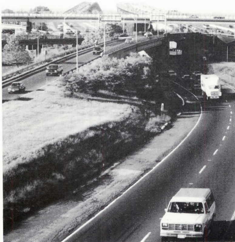
State and toll roads are often side by side like this juncture of I-287 Route 9 and the Garden State Parkway in Woodbridge. Therefore, coordination between the Department and the independent agencies is critical to efficient and safe movement of traffic.
