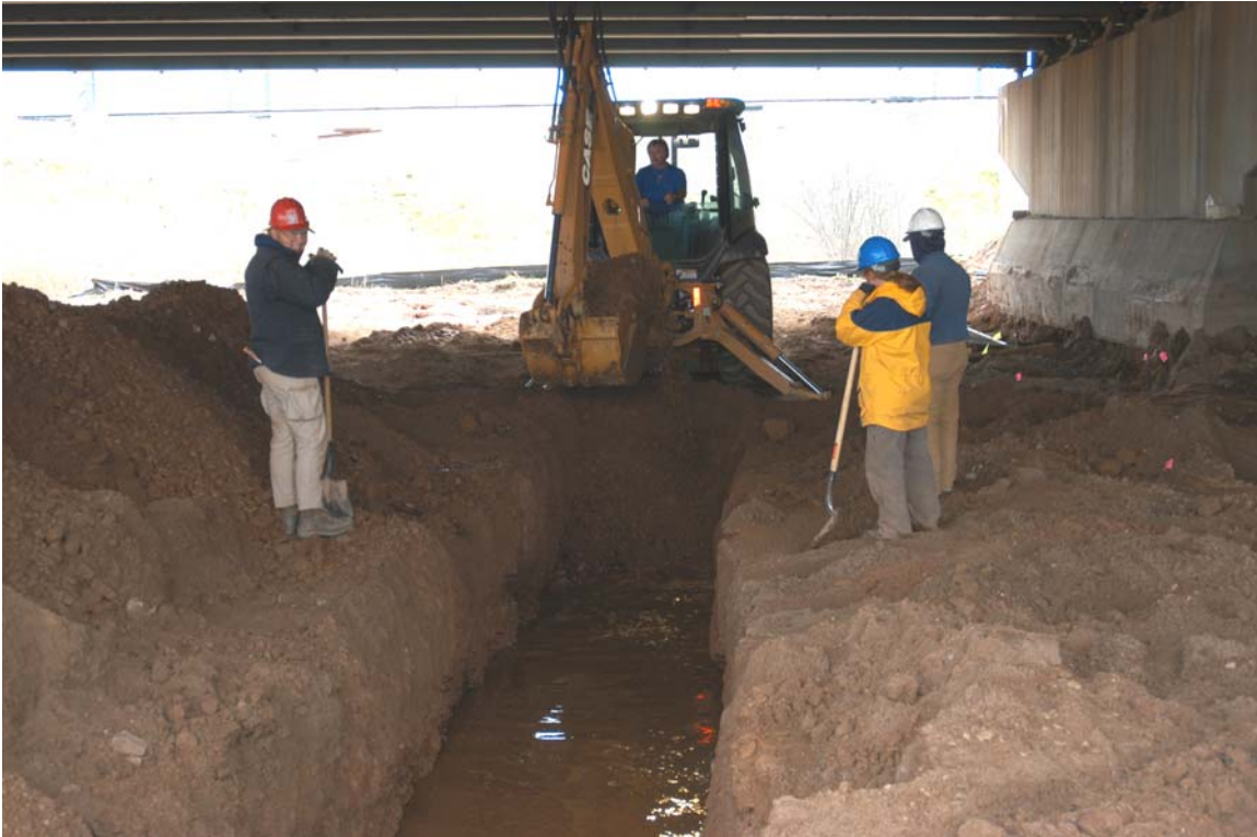
PLATE 7-15: Excavation of Exploratory Trench 2
