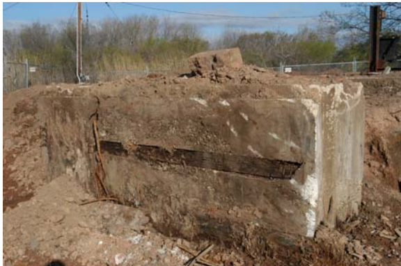
PLATE 7-1: Concrete Foundation Block from Billboard
