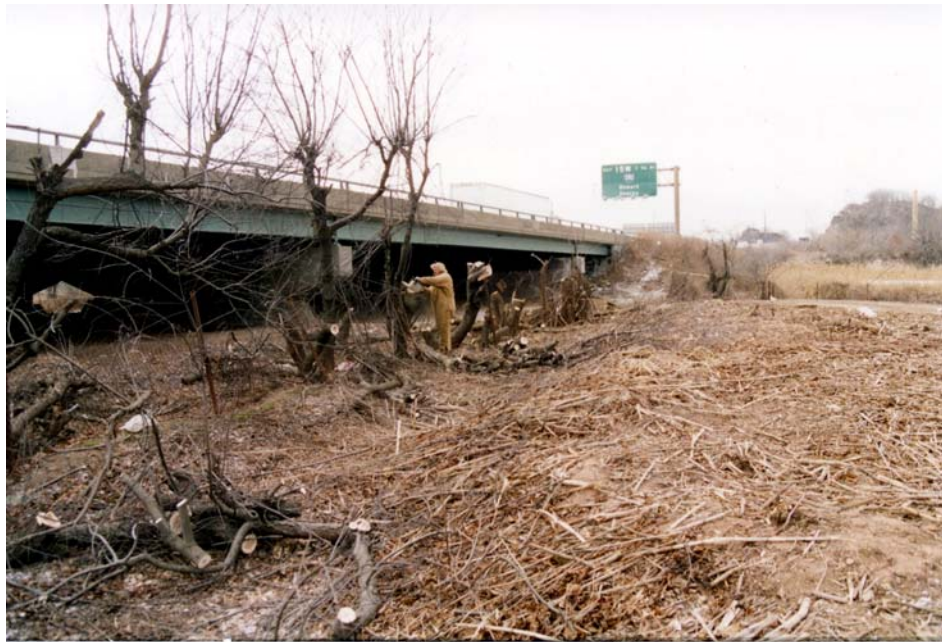
PLATE 5-7: Tree Clearing and Vegetation Removal at Potter's Field
