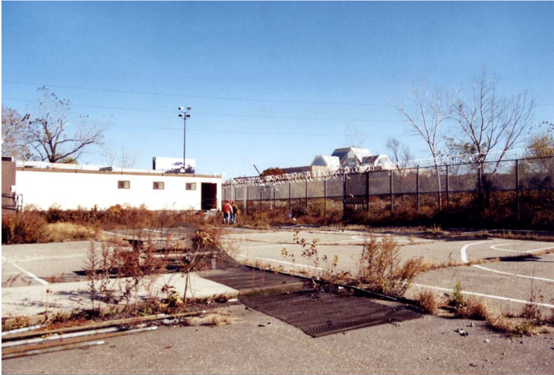
PLATE 5-10: Recreational Yard Area of Detention Center Covered With Macadam
