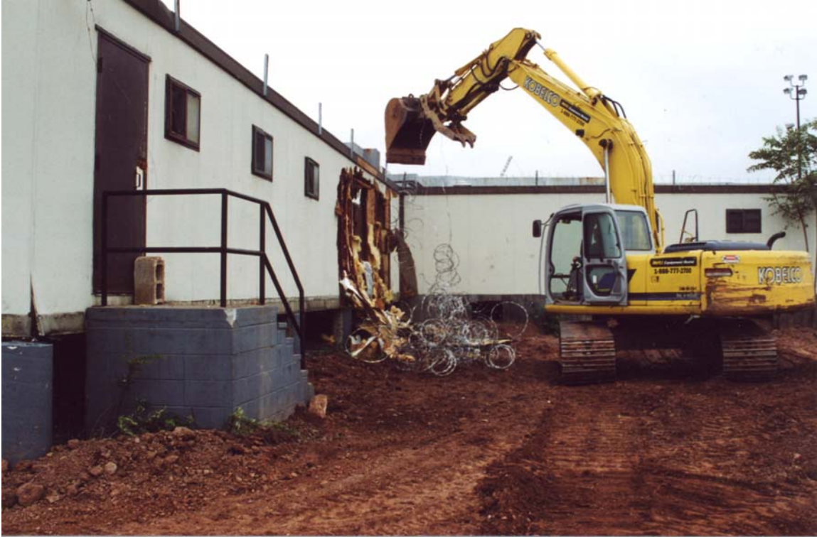
PLATE 7-5: Demolition of a Portion of Building B
