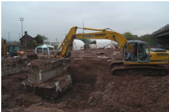
PLATE 7-3: Excavation Around Concrete Foundations
