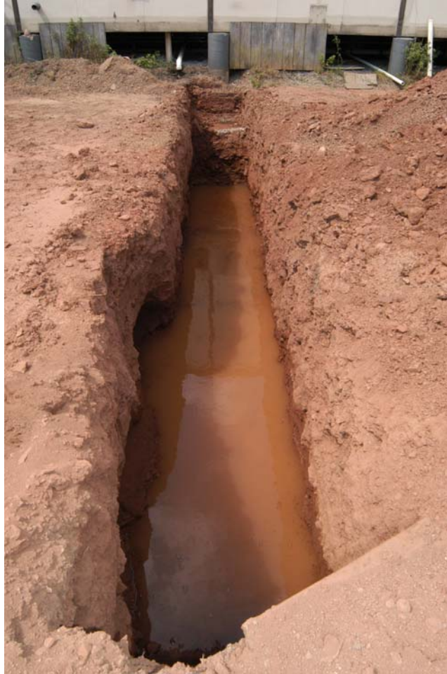
PLATE 7-17: Exploratory Trench 8 Adjacent to Building
