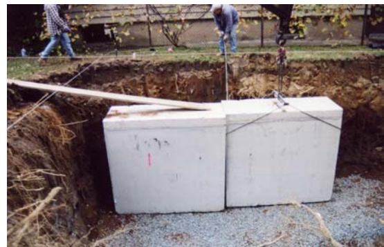
PLATE 10-4: Installation of Burial Vaults
