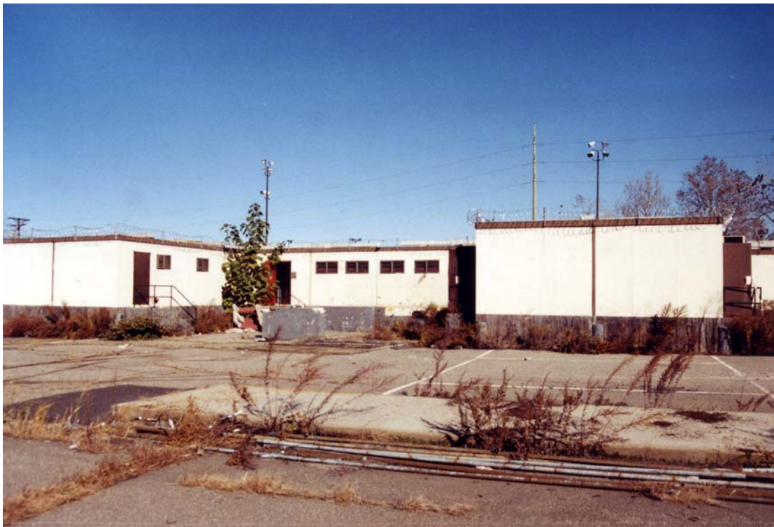
PLATE 5-11: General View of Abandoned Detention Center Building
