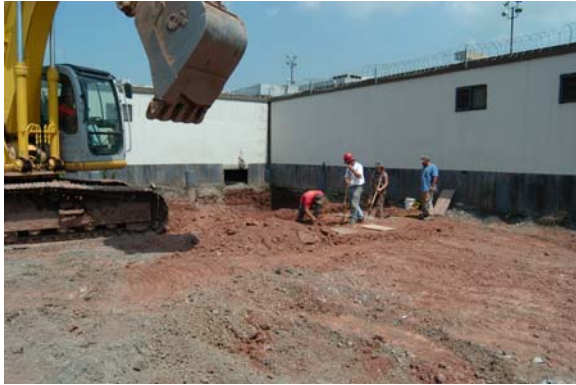
PLATE 7-30: Stripping Adjacent to Building B
