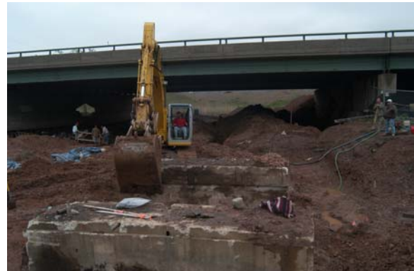
PLATE 7-2: Removal of Billboard Foundation Blocks
