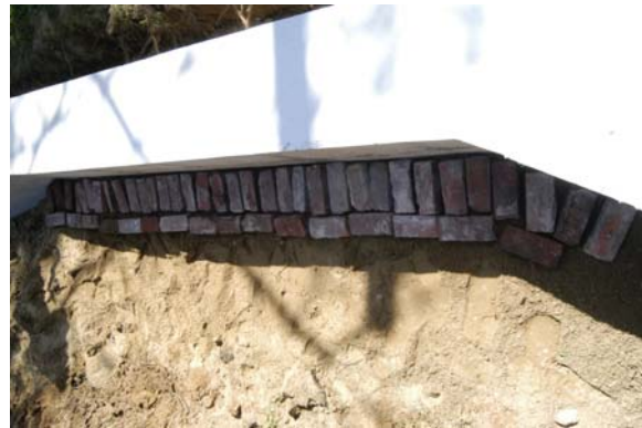
PLATE 10-11: Red Brick Embedded in Foundation of Memorial Monument
