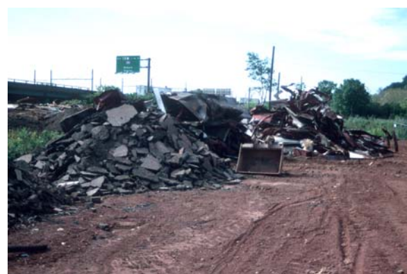
PLATE 5-27: Asphalt and Scrap Metal Debris
