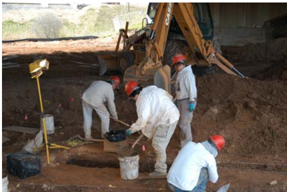
PLATE 7-13: Excavations Under Bridge
