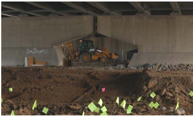
PLATE 7-11: Stripping Begins Under Turnpike Bridge
