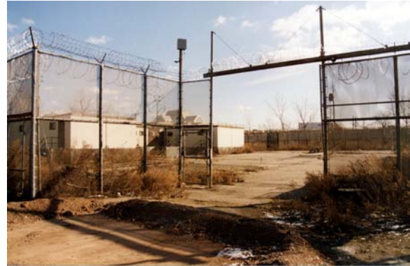
PLATE 5-9: Abandoned Detention Center
