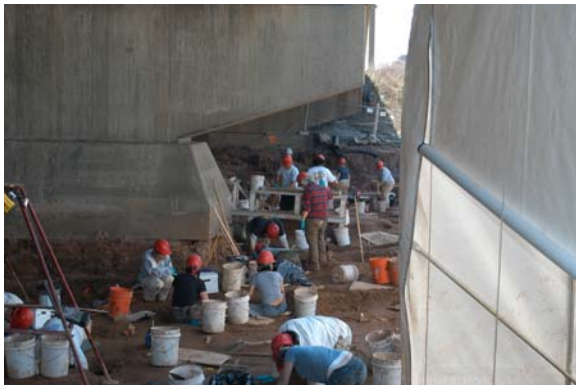
PLATE 5-33: Excavation and Screening
