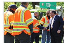
Route 80 Overpass Repair Project May 9, 2017
