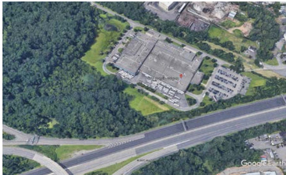
WAYNE BUS GARAGE
