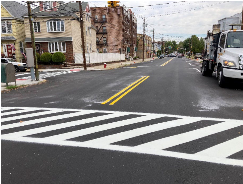
Bayonne City 2021 Roadway Improvements
