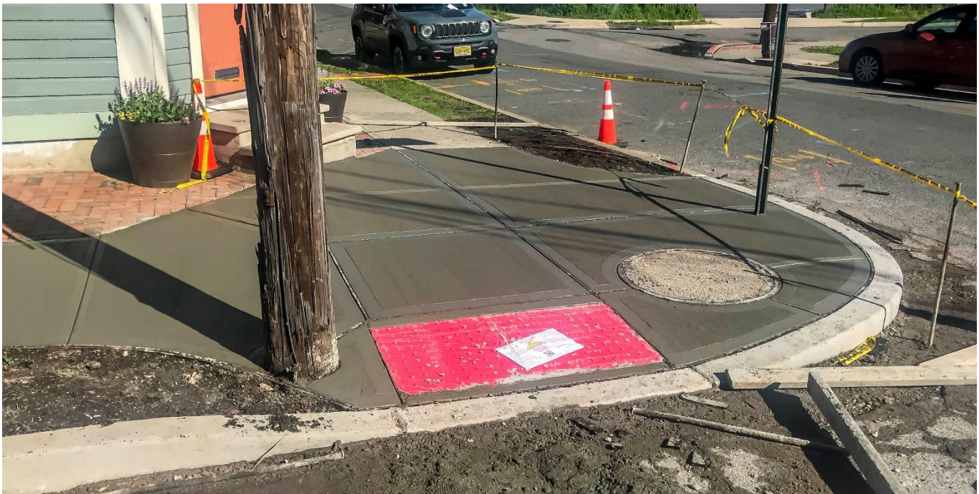
Orange City Various Street Paving Project
