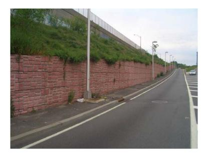
a wing wall under an overpass in Milltown. Various application and cleaning methods were utilized and documented. The picture above shows the first field location two years after the coating application.
