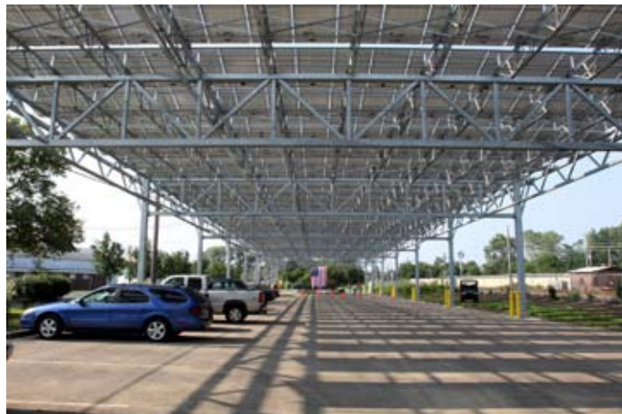
Sea Girt solar project covers a parking lot while saving the department money. Photo by Mark Olsen, DMAVA Public Affairs specialist.
