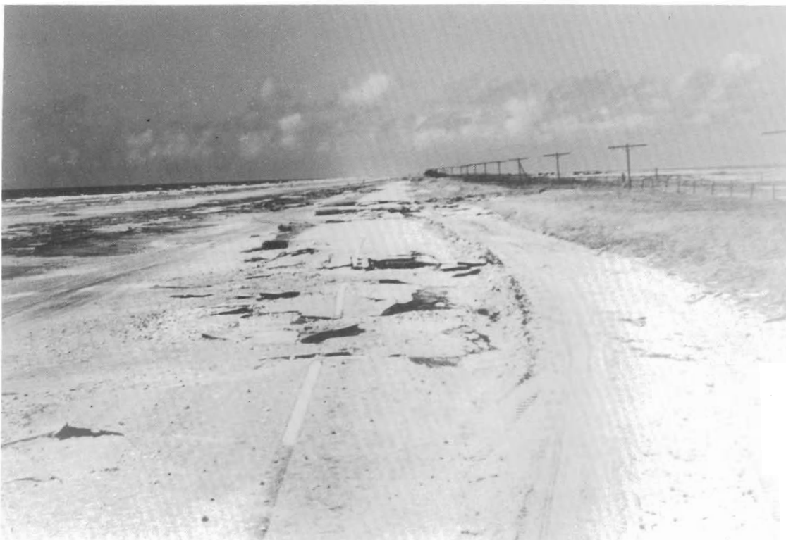
Texas Coastal Road Washed Out by Hurricane Carla
